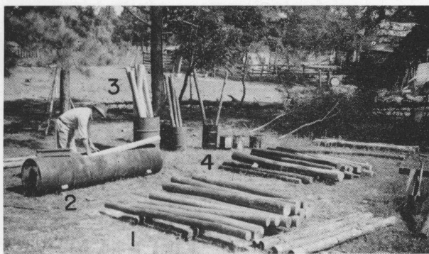
Figure 6. All the steps in treating insect-peeled posts are shown here: (1) untreated posts; (2) the posts are soaked full length in a vat of borax-boric acid or polybor; (3) after drying, they are sealed at ground ends by soaking in drums of heavy oil; (4) posts that have been treated and sealed.
