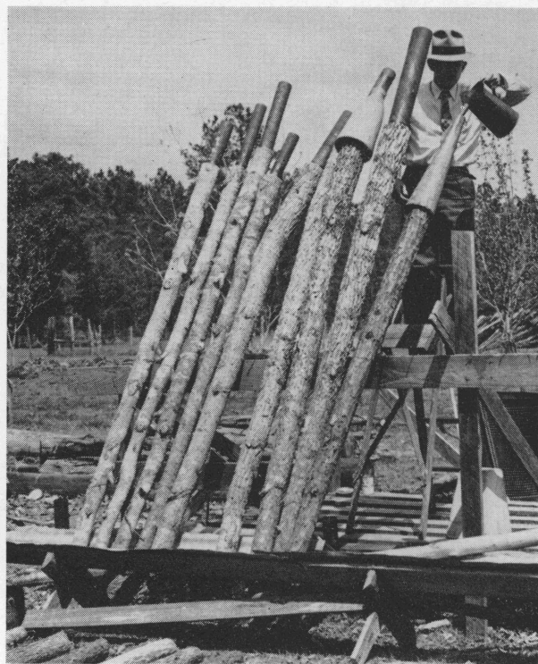
Figure 8. A waterborne preservative is measured into pipe and cone receptacles for end-flow treatment of these small posts. The sharpened pipes are cheaper to use since the cone receptacles require rubber gaskets.
