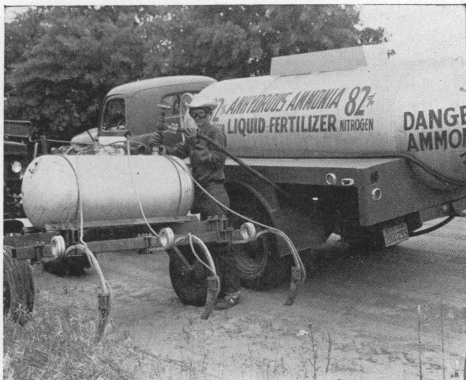
Equipment needed for applying anhydrous ammonia. (Courtesy of Tulsa Daily World.)
