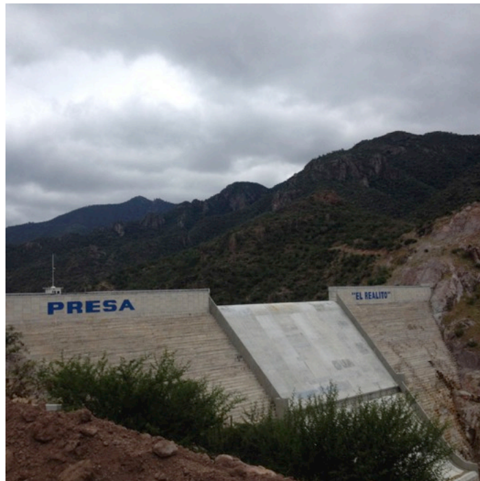
Figure 5.1 The Realito Dam. (Photo by the author)
