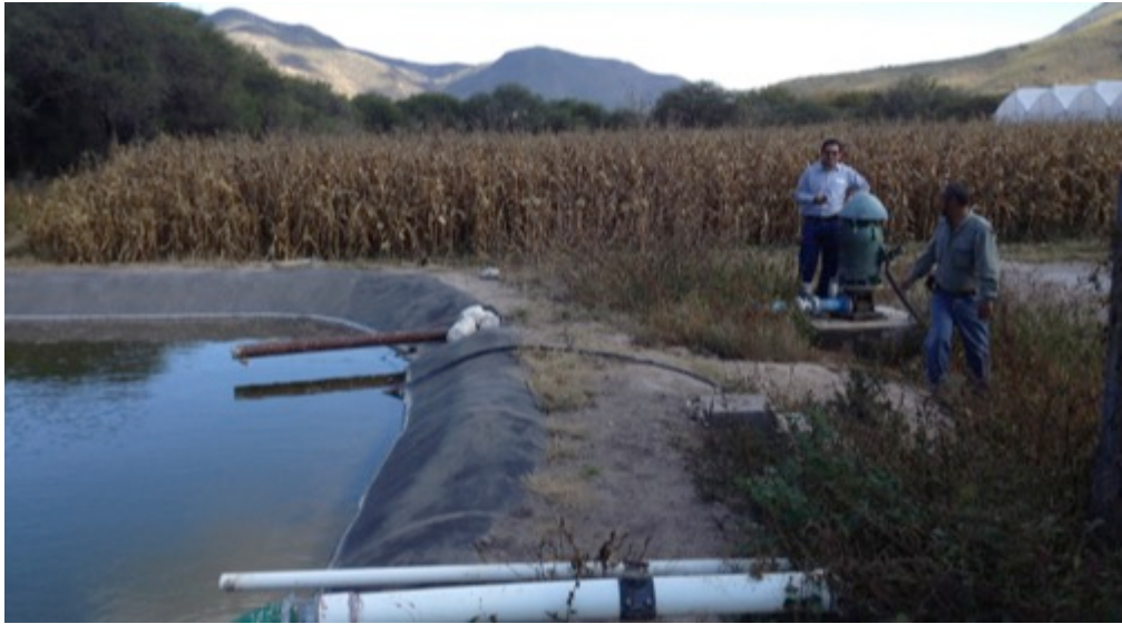
Figure 4.2 Reservoir storage of groundwater with pump. (Photo by the author)
