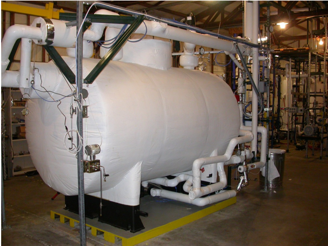
Figure 12: Completed Suppression Chamber and Nearby Plumbing
