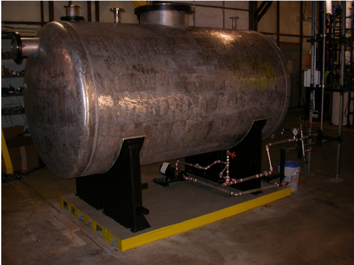
Figure 16: Suppression Chamber Analog During Facility Assembly
