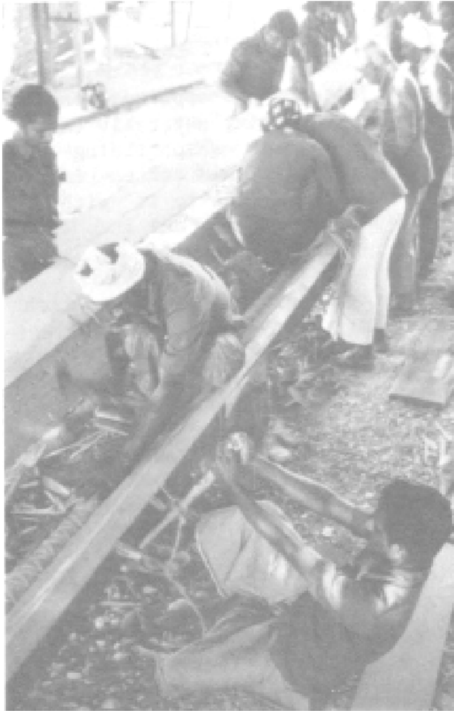
Figure 6.3: Agatti stitchers lacing the Omani Sohar (Severin 1985, 17.1).
