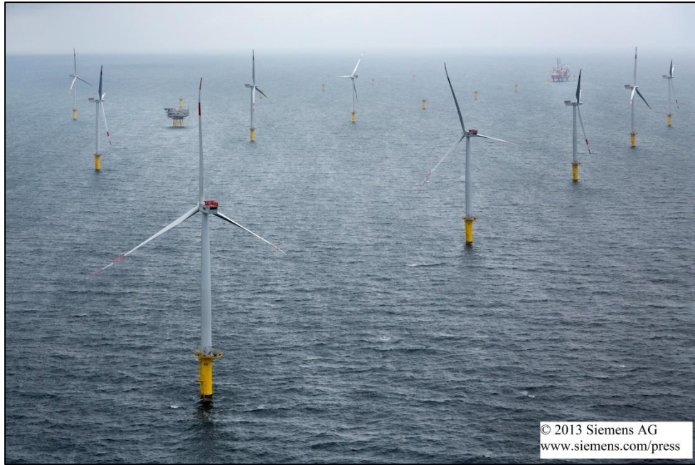
Figure 1-10 Riffgat offshore wind farm and offshore substation. Photo: Siemens AG 2013 [18]. Reused with courtesy of Siemens AG.
