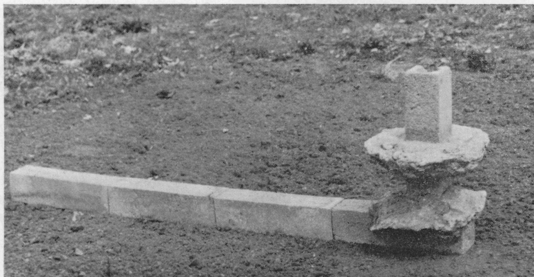
Feed pipe and tile line have been dug out of the ground to show how feed pipe joints were plastered.
