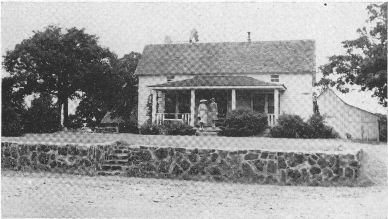
Grass on the lawn and a retaining wall help hold the soil at the Steve Arthur home, Tarrant County. The steps and wall of native stone are interesting features of this landscape.
