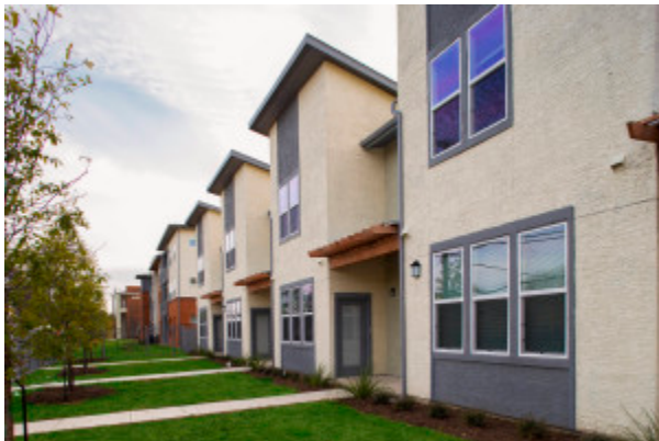
Figure 21 Affordable housing units in the Gardens at San Juan Square, San Antonio 1
