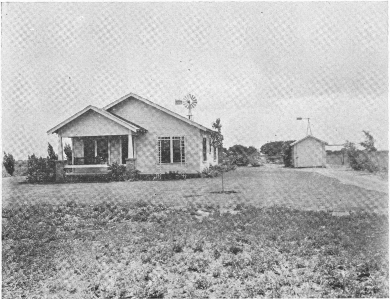
When cultivated crops were grown to the very threshold of this house the yard was marred by drifting hummocks of sand which persisted in forming. Now a planting of alfalfa entirely surrounds the homestead. The alfalfa stopped the forming of hummocks and stops much of the dust and mud which formerly reached the house.
