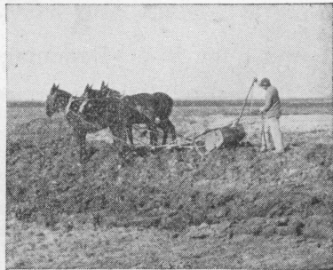
FIG. 12.—Making a fill where a terrace crosses a gully.
