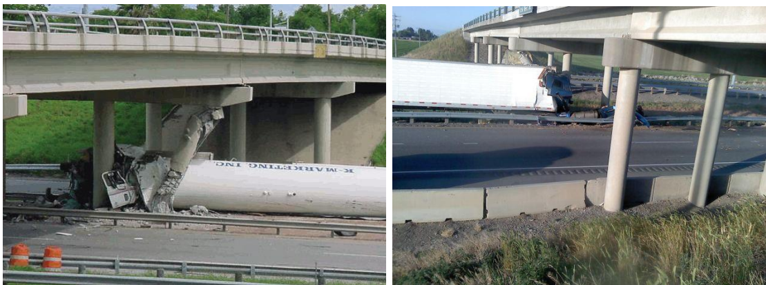
Figure 1-6: Bridge-vehicle crashes
