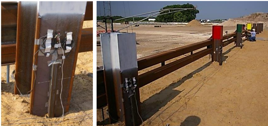
Figure 3-12: Instrumentations installed on the piles
