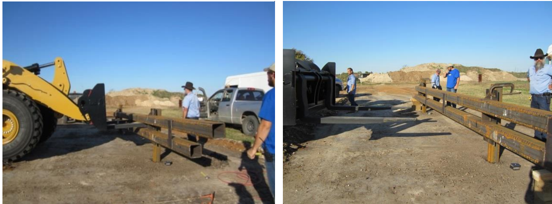
Figure 3-26: Installing the beams
