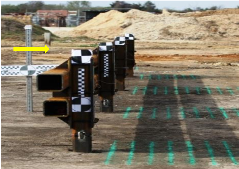
Figure 3-34: The barrier after installation
