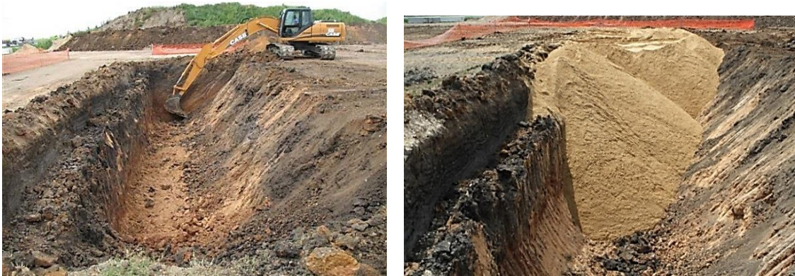
Figure 3-9: Loose sand ditch (Lim, 2011)
