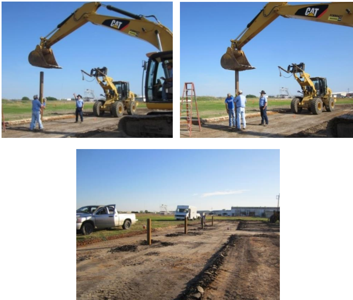
Figure 3-25: Pile driving into the hard clay
