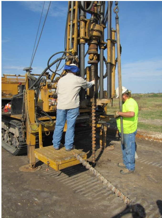
Figure 3-36: Standard Penetration Testing and sampling
