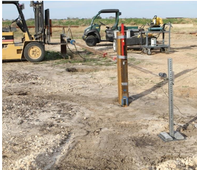
Figure 3-20: The static test installation
