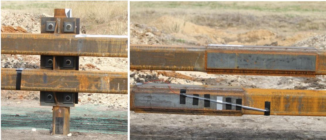
Figure 3-33: Anchor bolts (left), the plates welded to beams (right)
