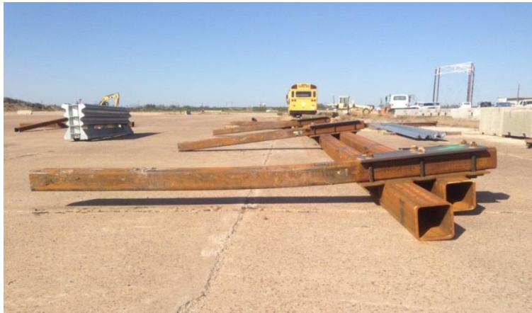
Figure 3-55: Piles after testing
