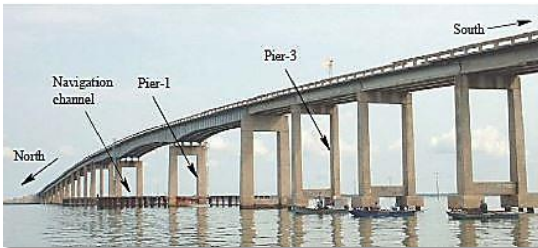
Figure 2-2: The St. George Island causeway bridge
