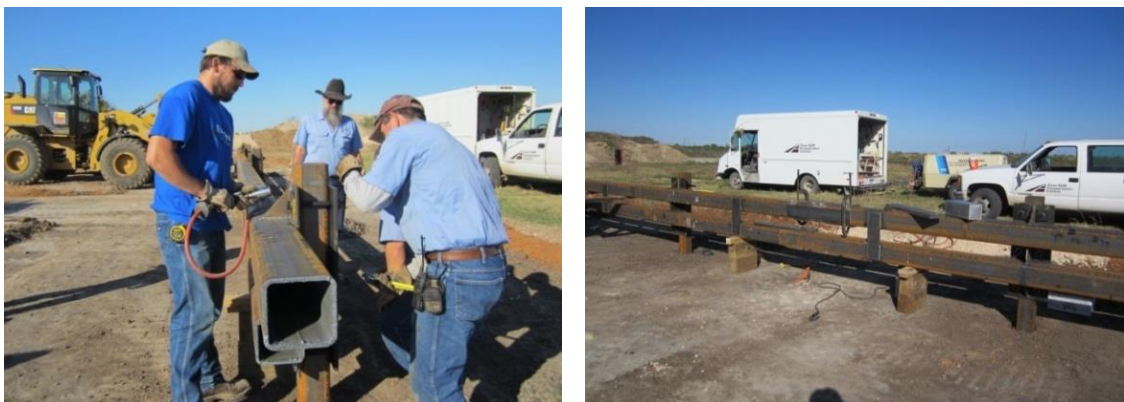
Figure 3-27: Connections installations using bolts and welding
