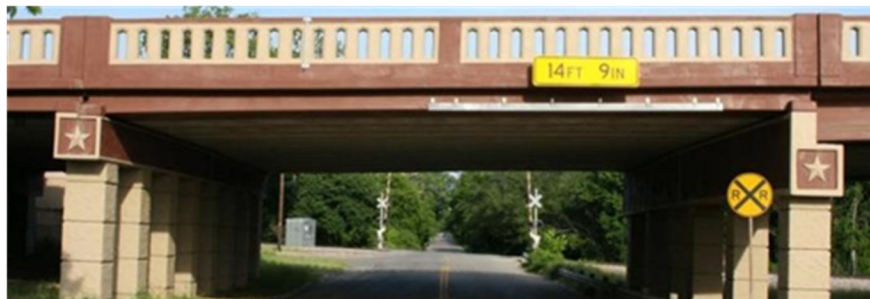
(d) US 69 Bridge Looking West along Day Street, Denison, Texas
