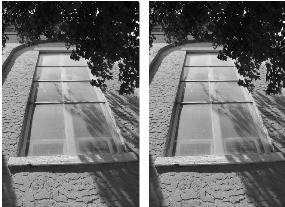
FIGURE 61. Image of protective plexiglas panels on the exterior of the building. (Photograph by the author)
