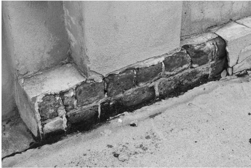
FIGURE 55. Image of stucco finish and exposed brick. (Photograph by the author)
