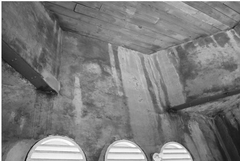
FIGURE 71. Image of the interior of the existing steeple. (Photograph by the author)
