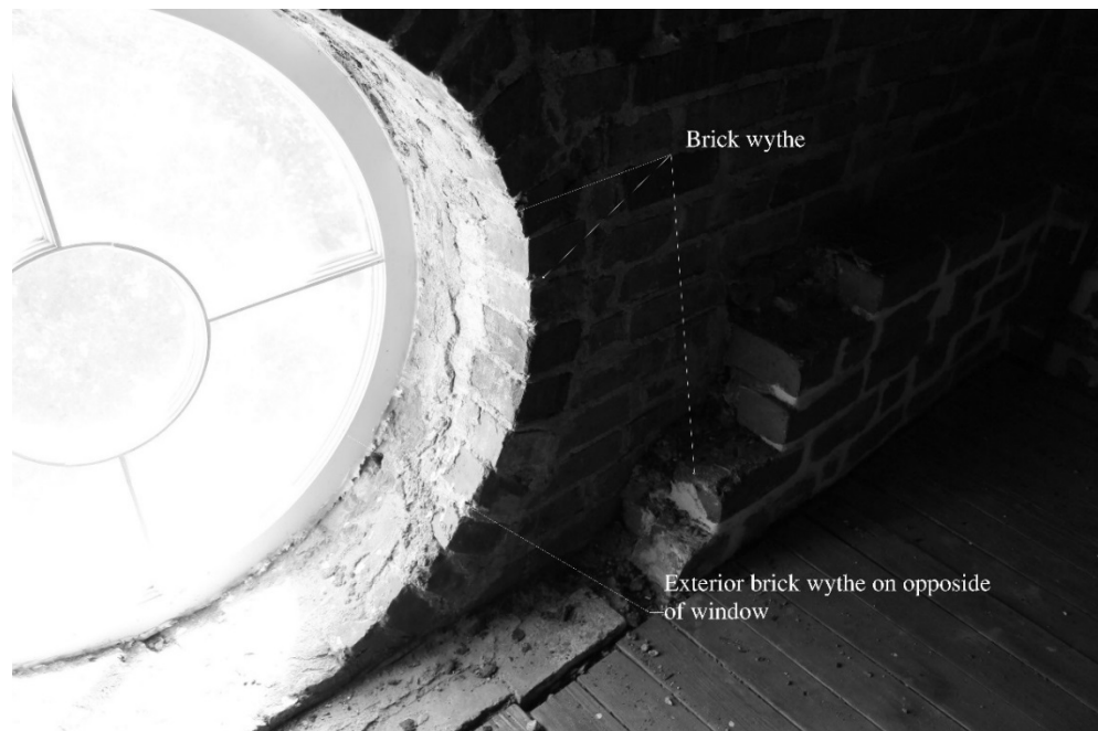
FIGURE 35. Image of a multi brick wythe wall in the bell tower of the First African Baptist Church (Photograph by the author)
