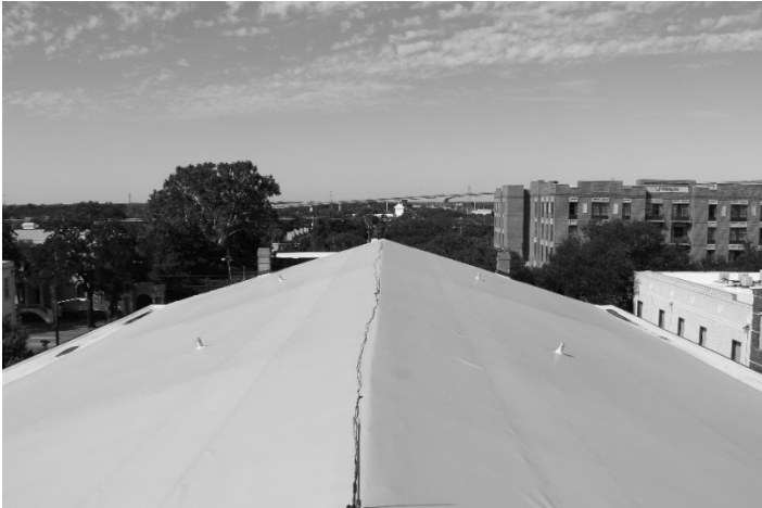
FIGURE 41. Image of the finished roof system (Photograph by the author)
