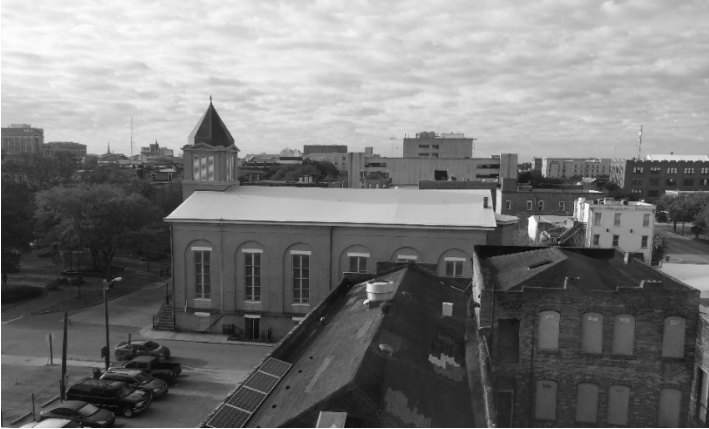
FIGURE 40. Image of the finished roof system. (Photograph by the author)
