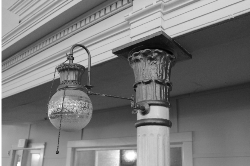
FIGURE 79. Image of gas light fixture in the sanctuary. (Photograph by the author)
