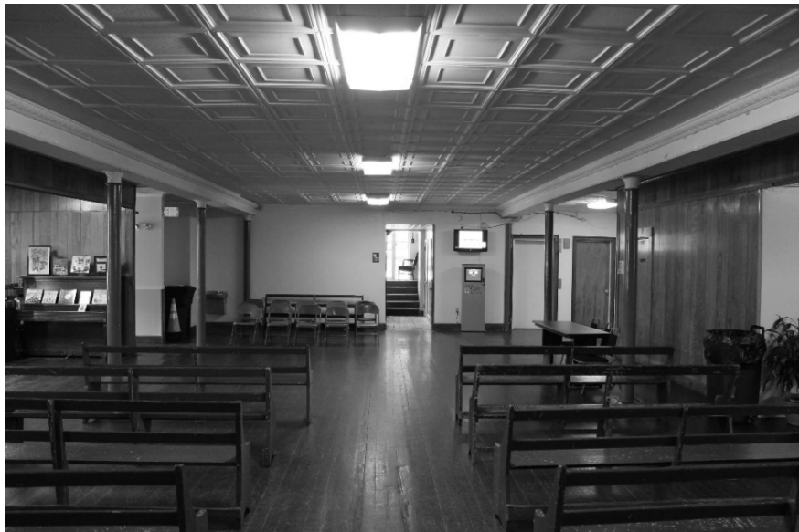
FIGURE 36. Image of the pipe columns in the Fellowship Hall of the First African Baptist Church. (Photograph by the author).
