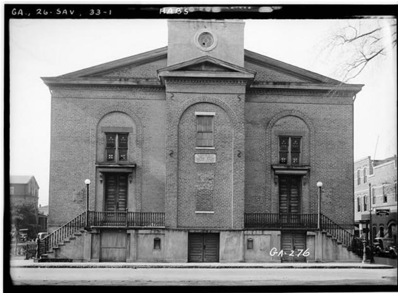
FIGURE 52. Image of church building from the Historic American Building Survey, circa 1936.
