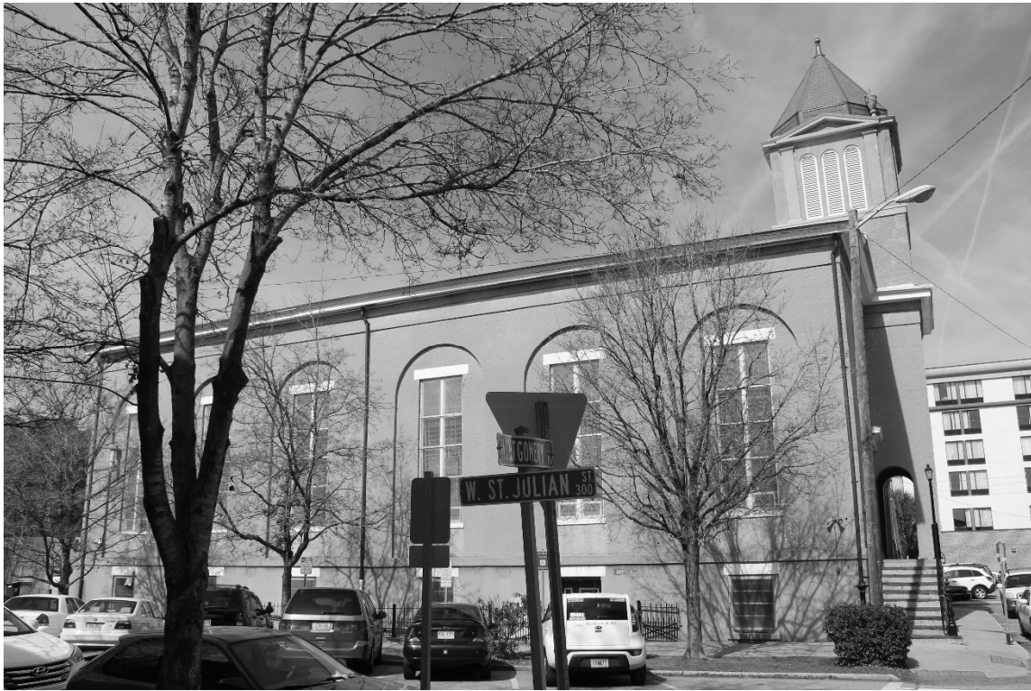
FIGURE 3. South elevation of the First African Baptist Church (Photograph by the author)
