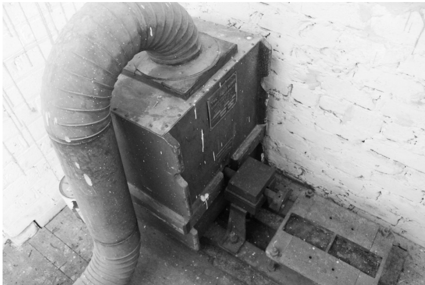
FIGURE 74. Image of kinetic organ blower located in the bell tower of the building. (Photograph by the author)
