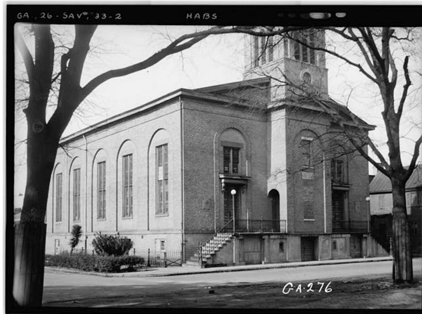
FIGURE 51. Image of church building from the Historic American Building Survey, circa 1936.
