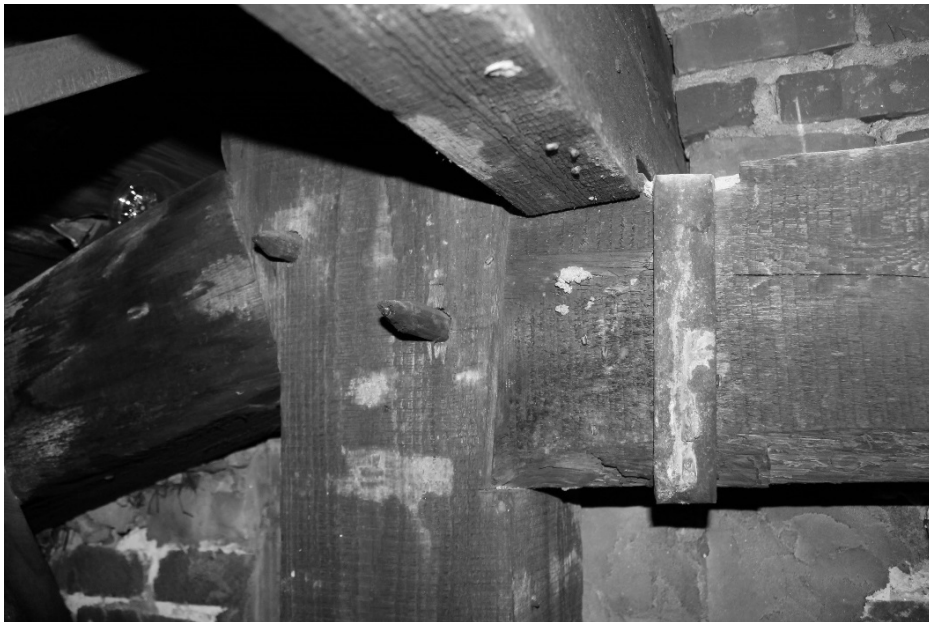
FIGURE 48. Image of tapered wooden pins (nails). (Photograph by the author)
