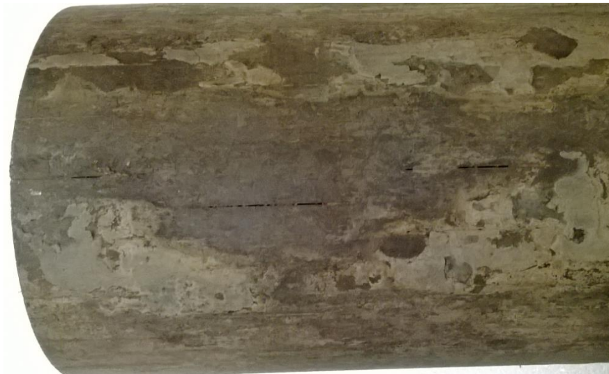
Figure 2.43 – Bottom part of liner #3
