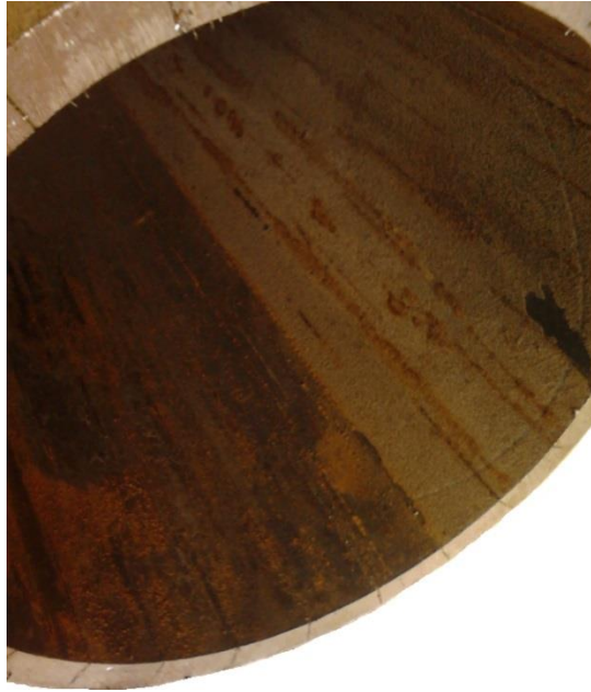
Figure 2.56 – Inner surface of liner #3
