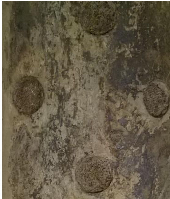
Figure 2.25 – Section of liner #2 with blocked openings
