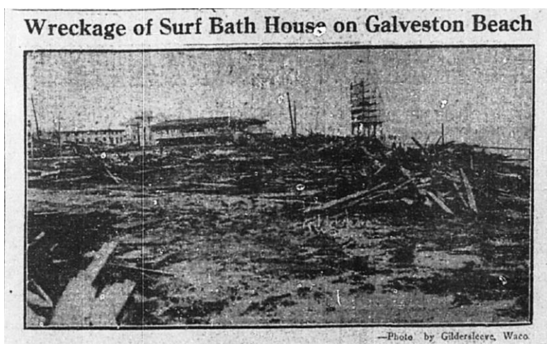
Fig. 17. “Wreckage of Surf Bath House on Galveston Beach,” photograph by Gildersleeve, Waco, Dallas Morning News , August 22, 1915, p 6.
