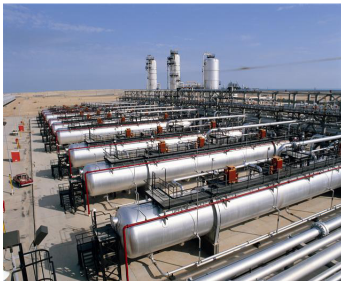
Figure 1.2: Gas-Oil Separation Plants (GOSP) facility at Murjan, Saudi Arabia. (courtesy: www.poonglim.co.kr ).
