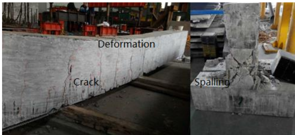
Figure I.1 Concept of damage (Federal Highway Administration, 2007)
