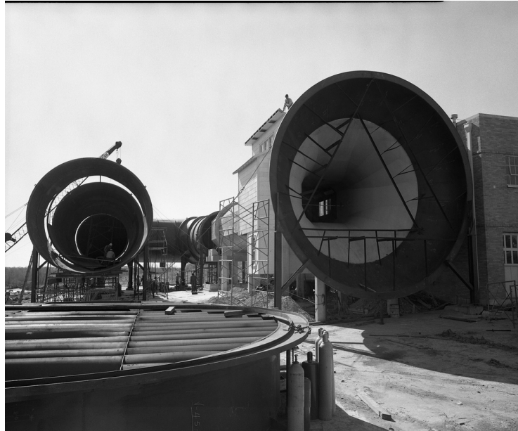
Figure 1.1: LSWT closed-circuit construction c.1958 [1][2]
