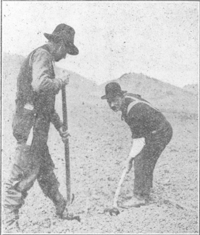
Digging Hole in such a way that locating stake will be in center of hole.
