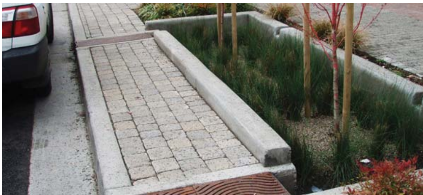
Figure 7-16 Stormwater Planter xvi
