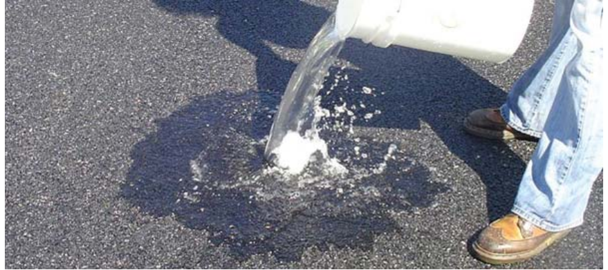
Figure 7-13 Pervious Paving xiii
