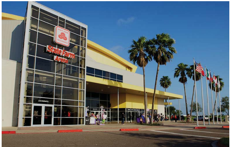
Figure 5-1 State Farm Arena i
