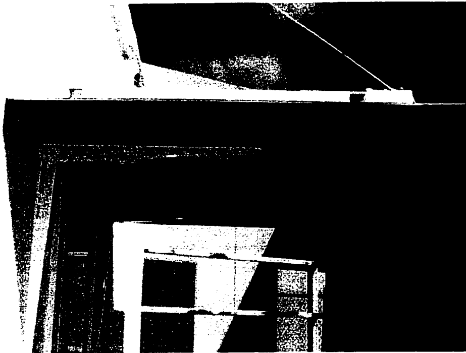
Figure A.19 Overhang Shading Device View from Below. The window aperture is to the left of the overhang.
