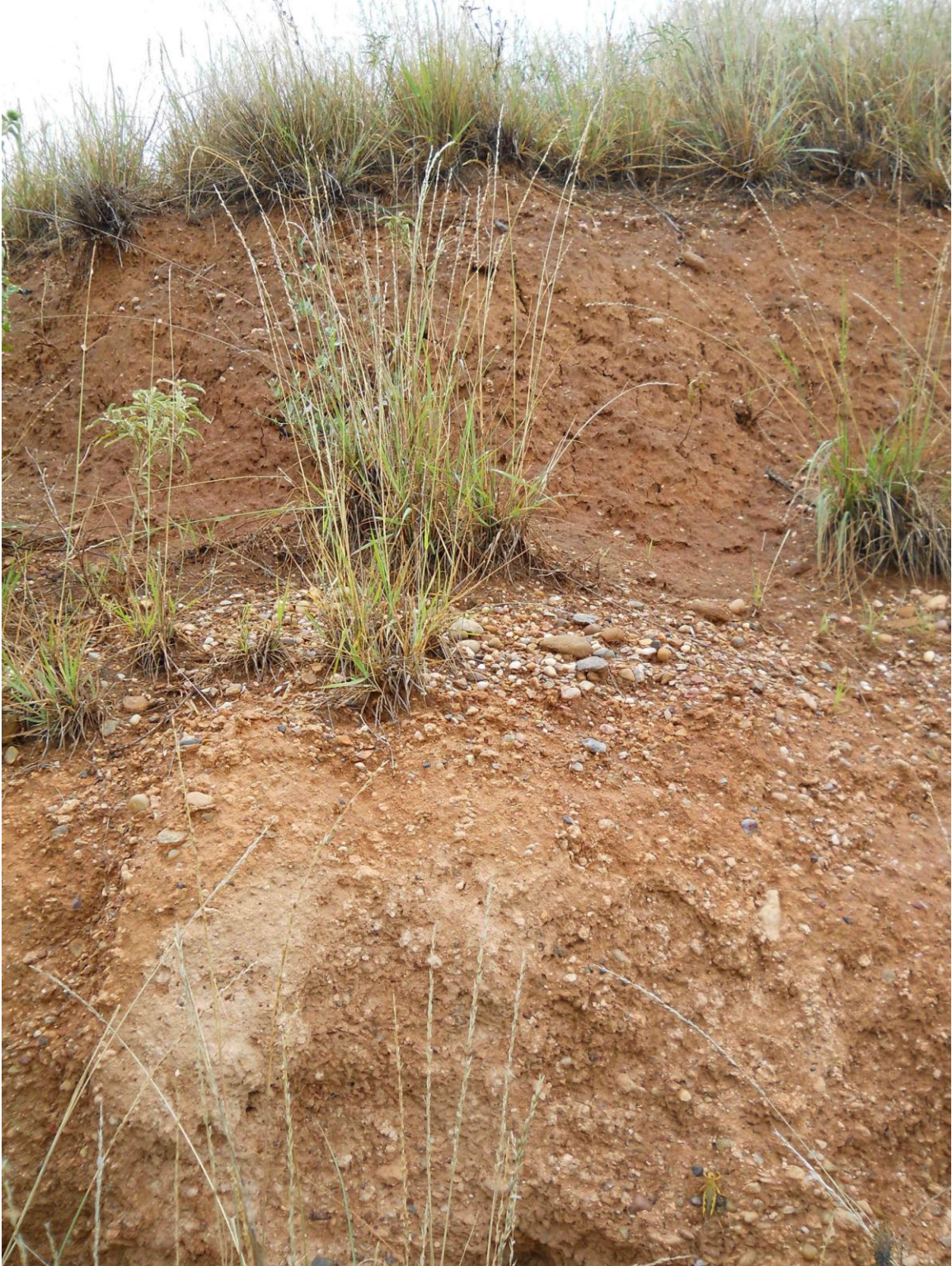
Profile of Exposed Bank at Area A
