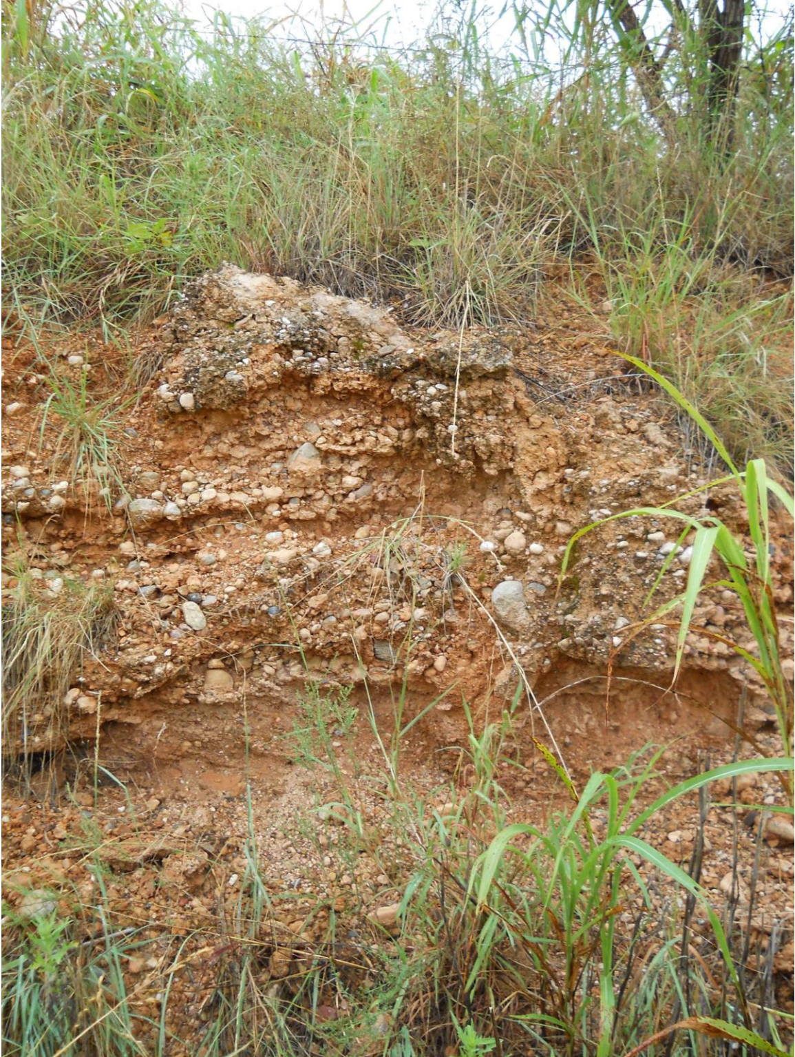
Profile of Exposed Bank at Area A
