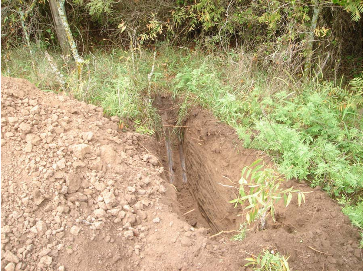
Area 1. Backhoe Trench 1 (during excavation)
