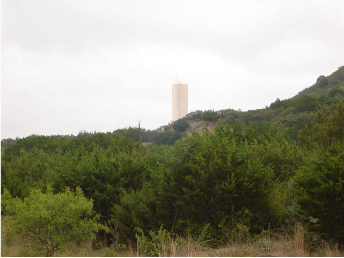
Area 4. View of Existing Water Storage Tank on Slope of Mesa
