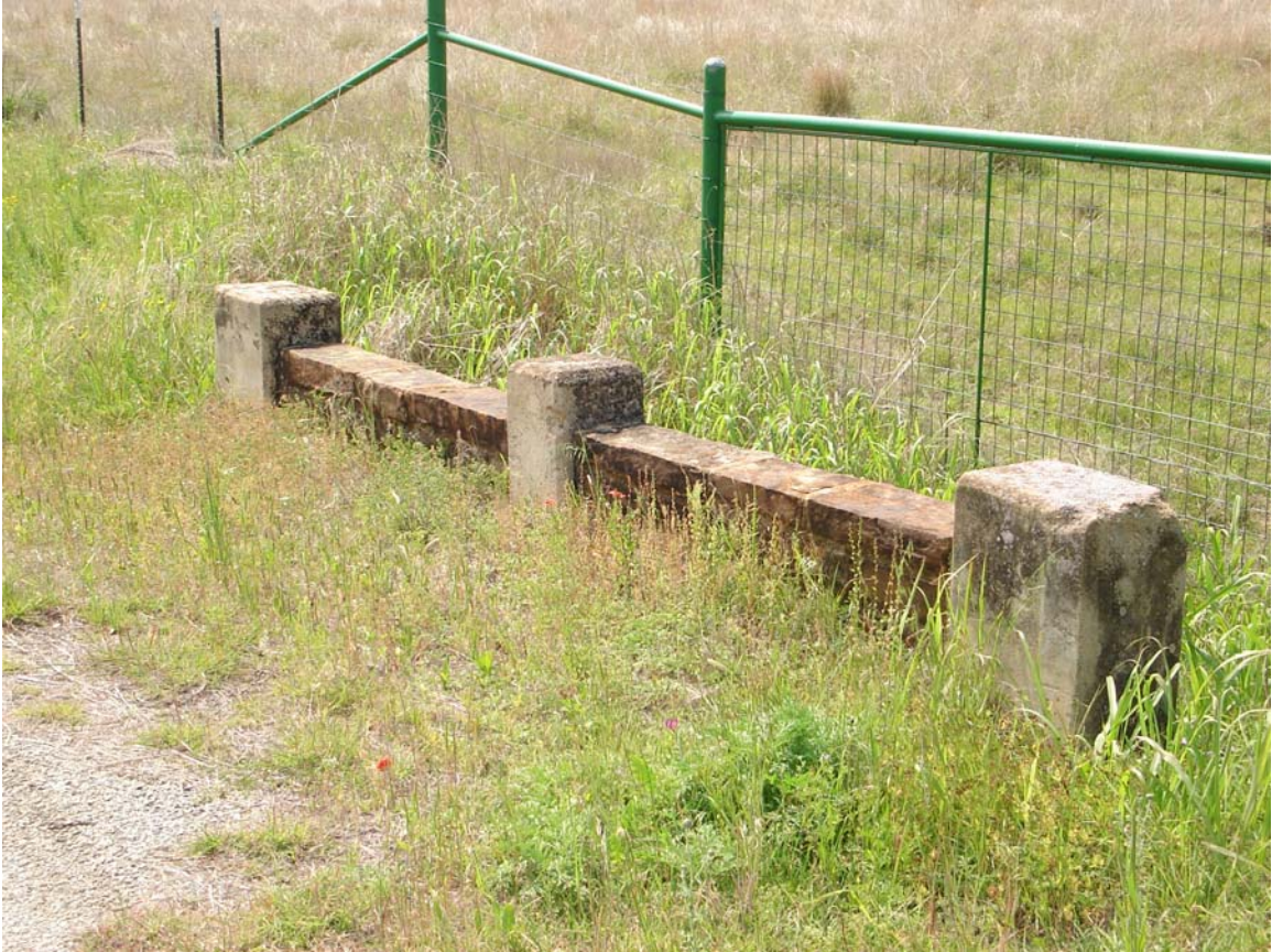
Low Water Crossing West of Creek
