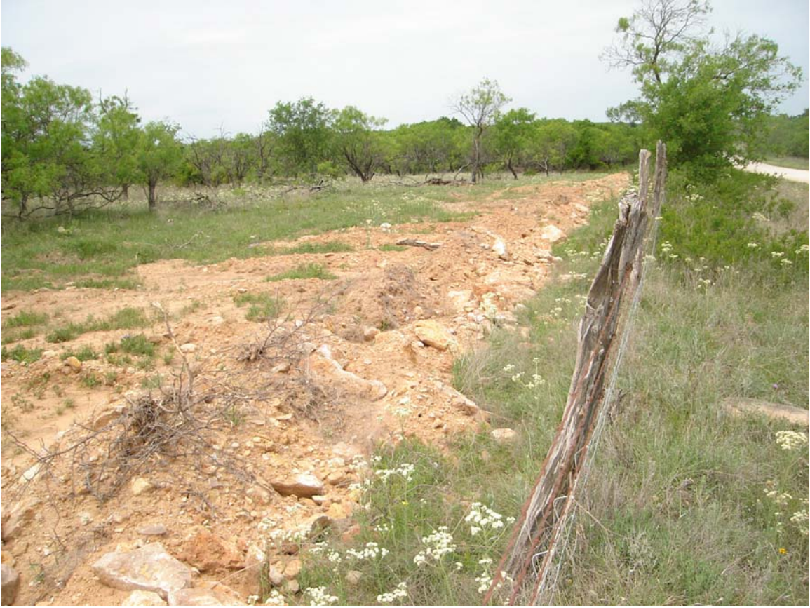
Figure 4. Disturbance along County Road 118
