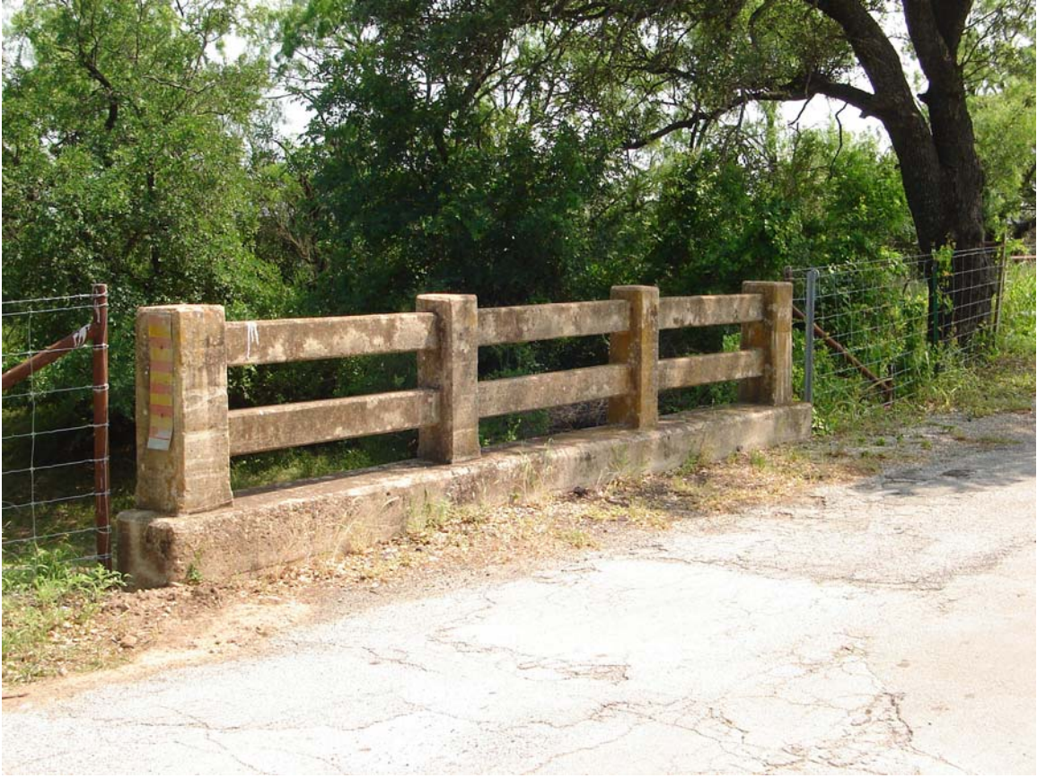
Bridge Crossing at Rough Creek
