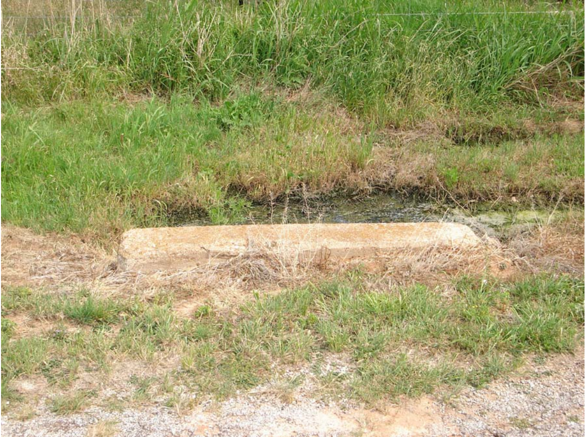
Low Water Crossing East of Creek
