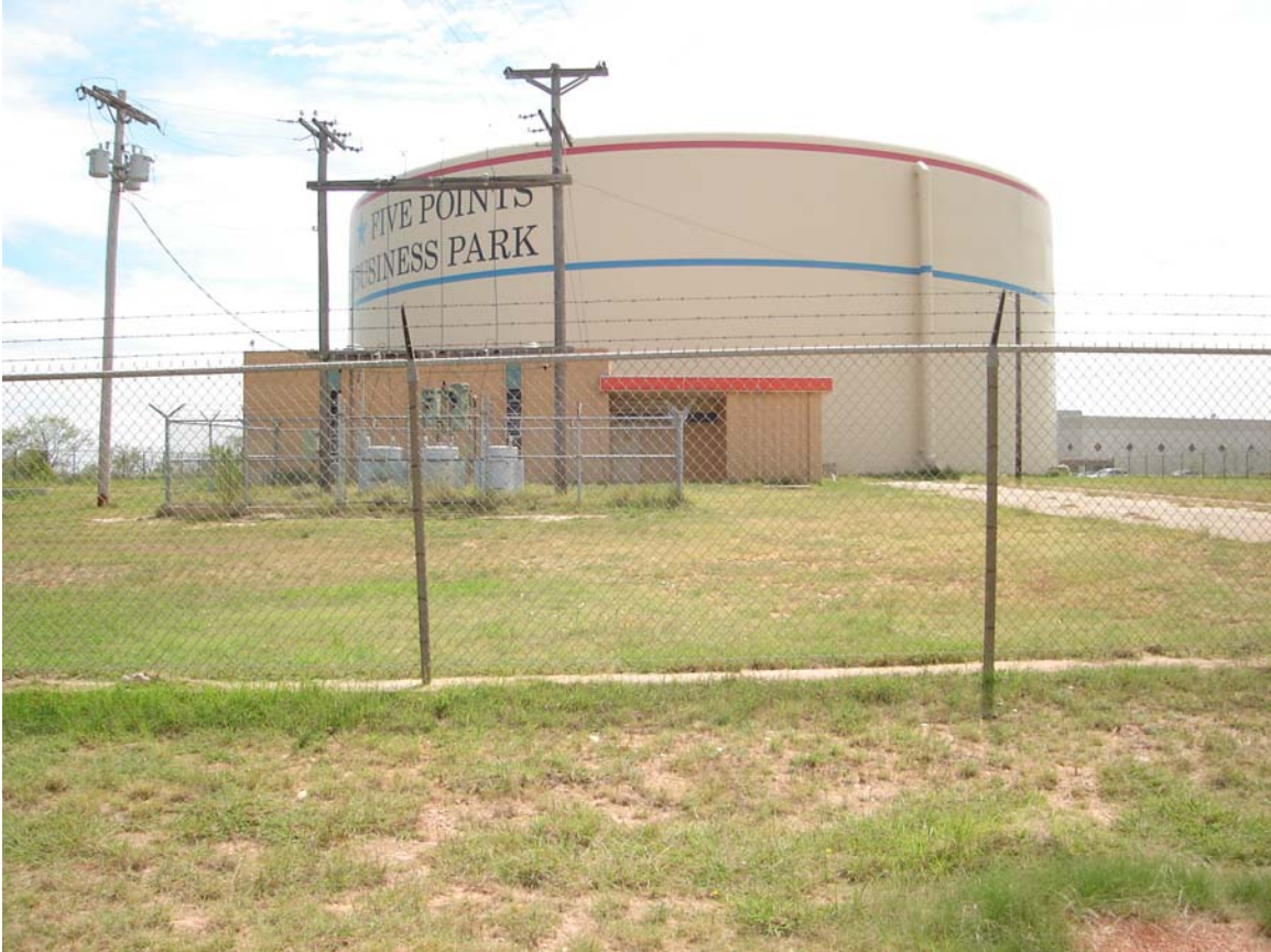
Figure 4. Existing Pump Station (looking south)
