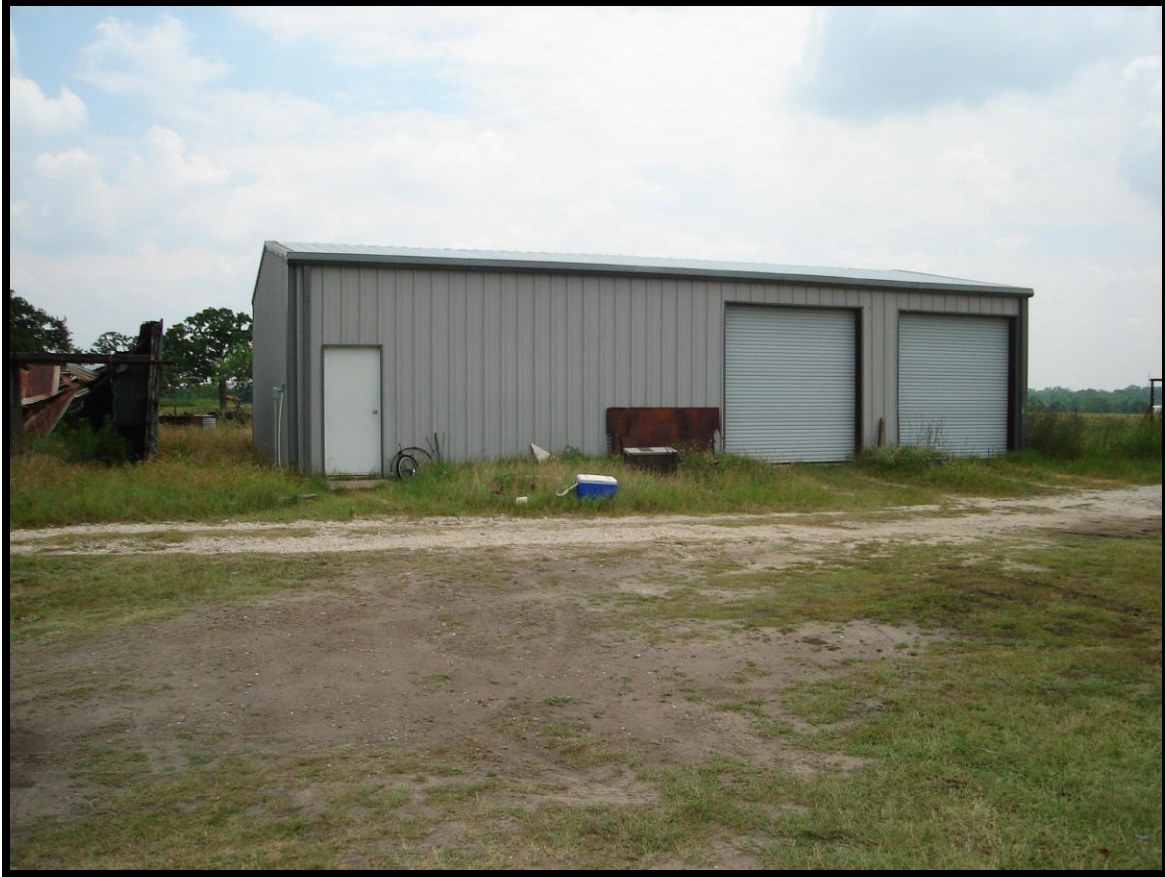
Structure G (modern metal building)
