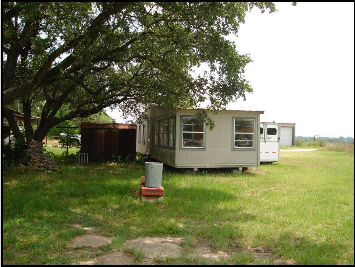
Structure B (unoccupied mobile home)
