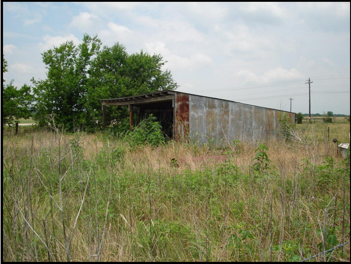
Structure D (pole barn)
