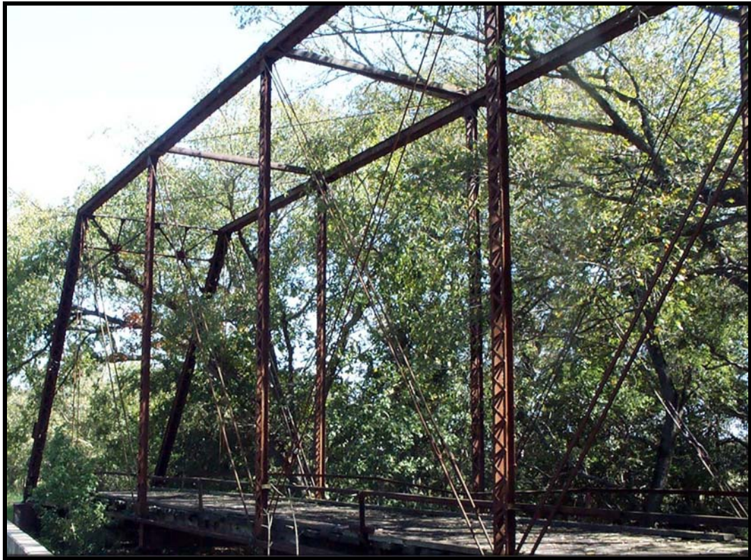
Figure 3. Plum Creek Through Truss Bridge (41CW91)
