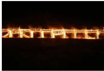
Figure 19. A portion of the international rail bridge between Presidio and Ojinaga was burned in February 2008. Arson was suspected as the cause of the blaze that destroyed the bridge.
