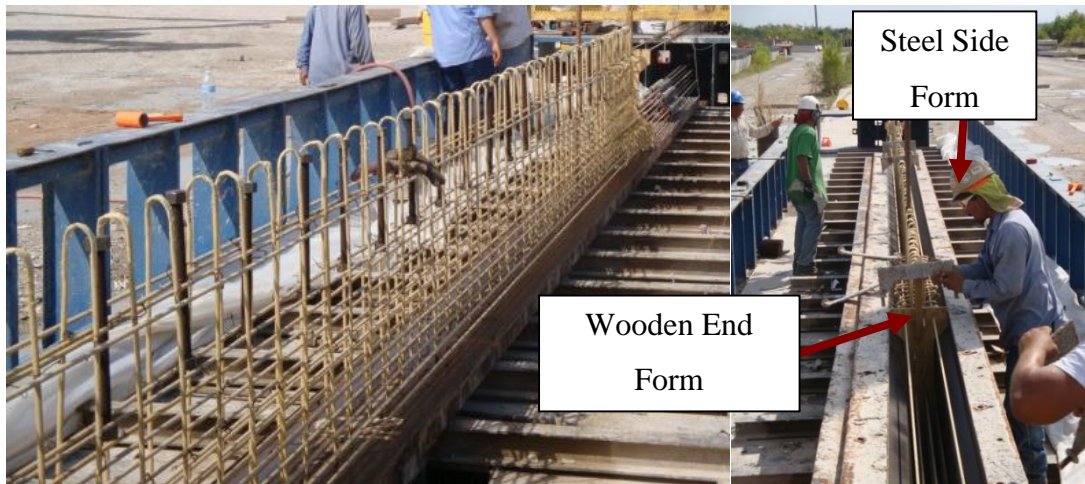
Figure 4-5. Girder Formwork and Reinforcement.
