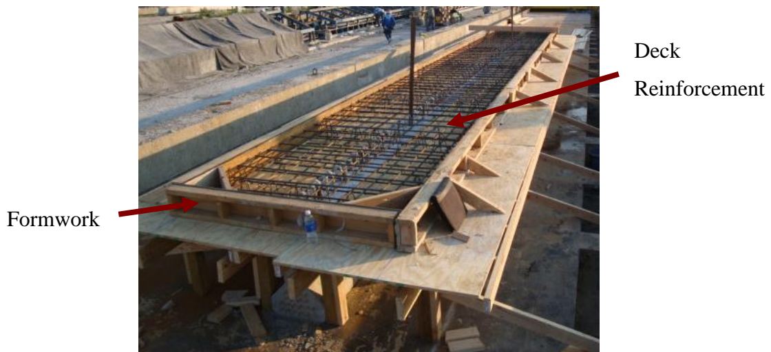
Figure 4-7. Deck Formwork and Reinforcement.
