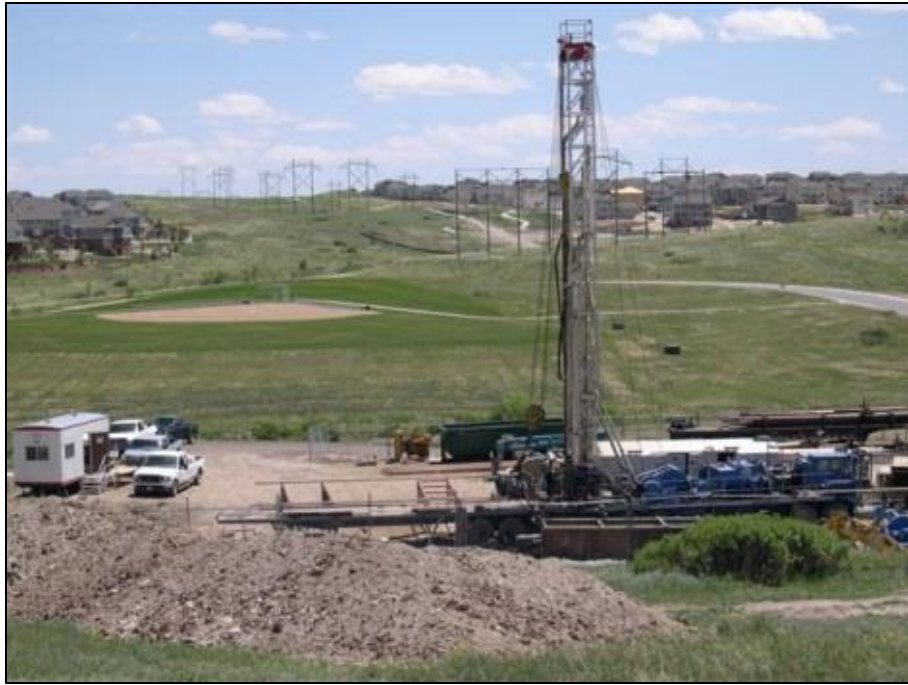
Figure 28. Castle Pines North Municipal District directional groundwater well rig. Reprinted from Jehn-Dellaport (2013).
