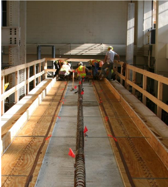
(a) Finished formwork
