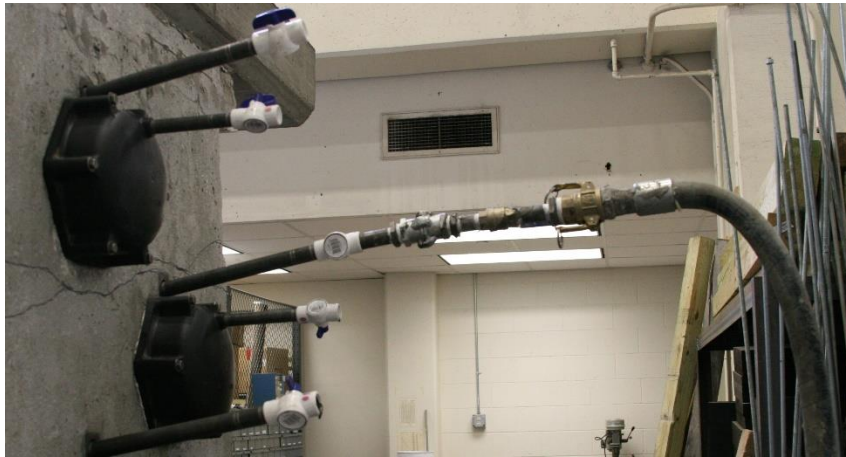
(c) Pressure grouting the ducts
