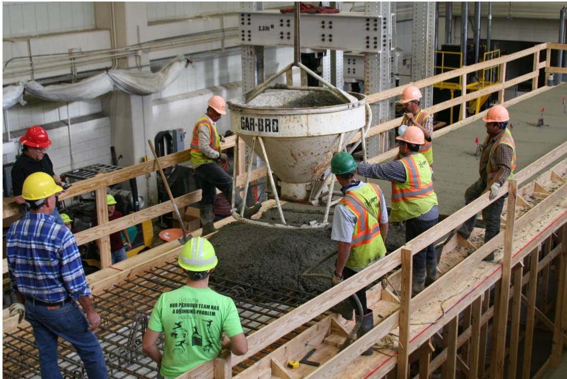
(c) Casting of the deck
