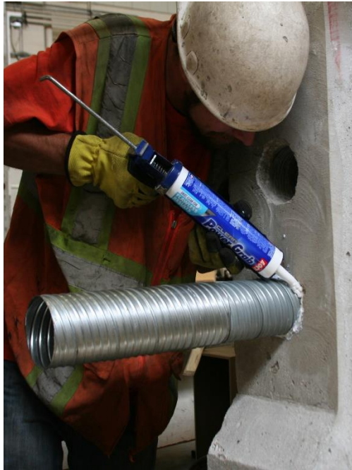
(a) Placing bottom duct
