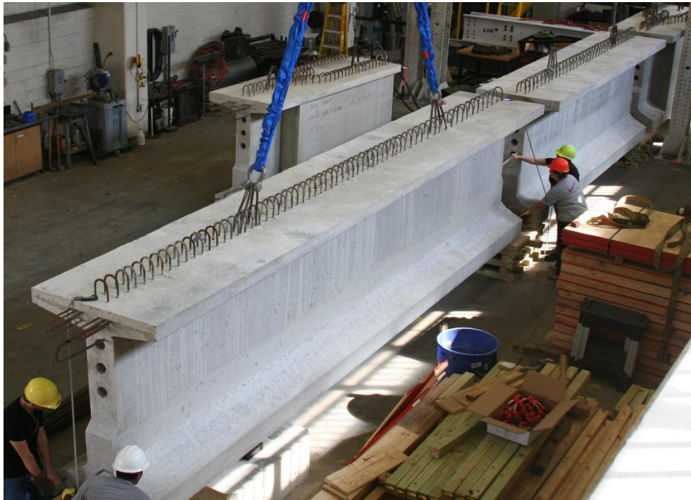
(a) Setting the second segment
