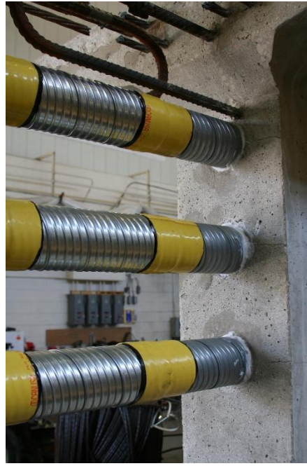
(b) Ducts placed and sealed
