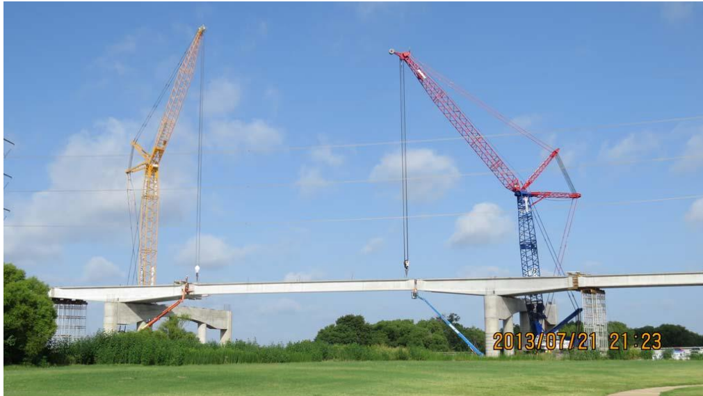
(a) Placing the drop-in segment within Span 11
