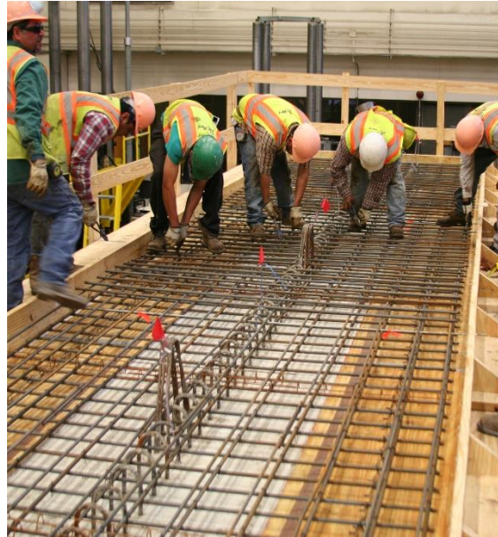
(b) Installation of deck reinforcement
