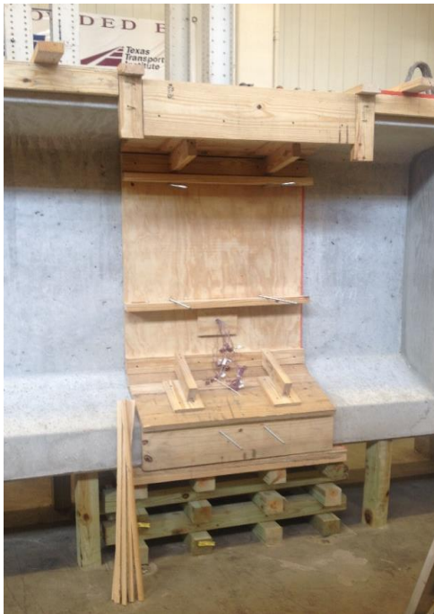
(a) Splice formwork
