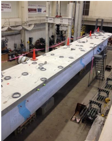
(a) Surface strain gages on top of the deck
