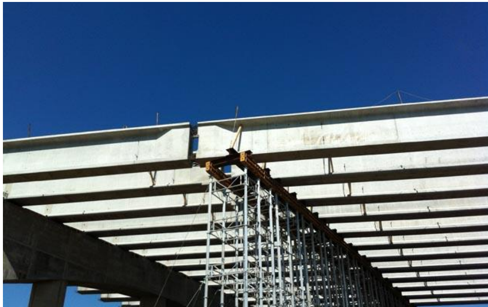
(b) Shore towers on back spans
