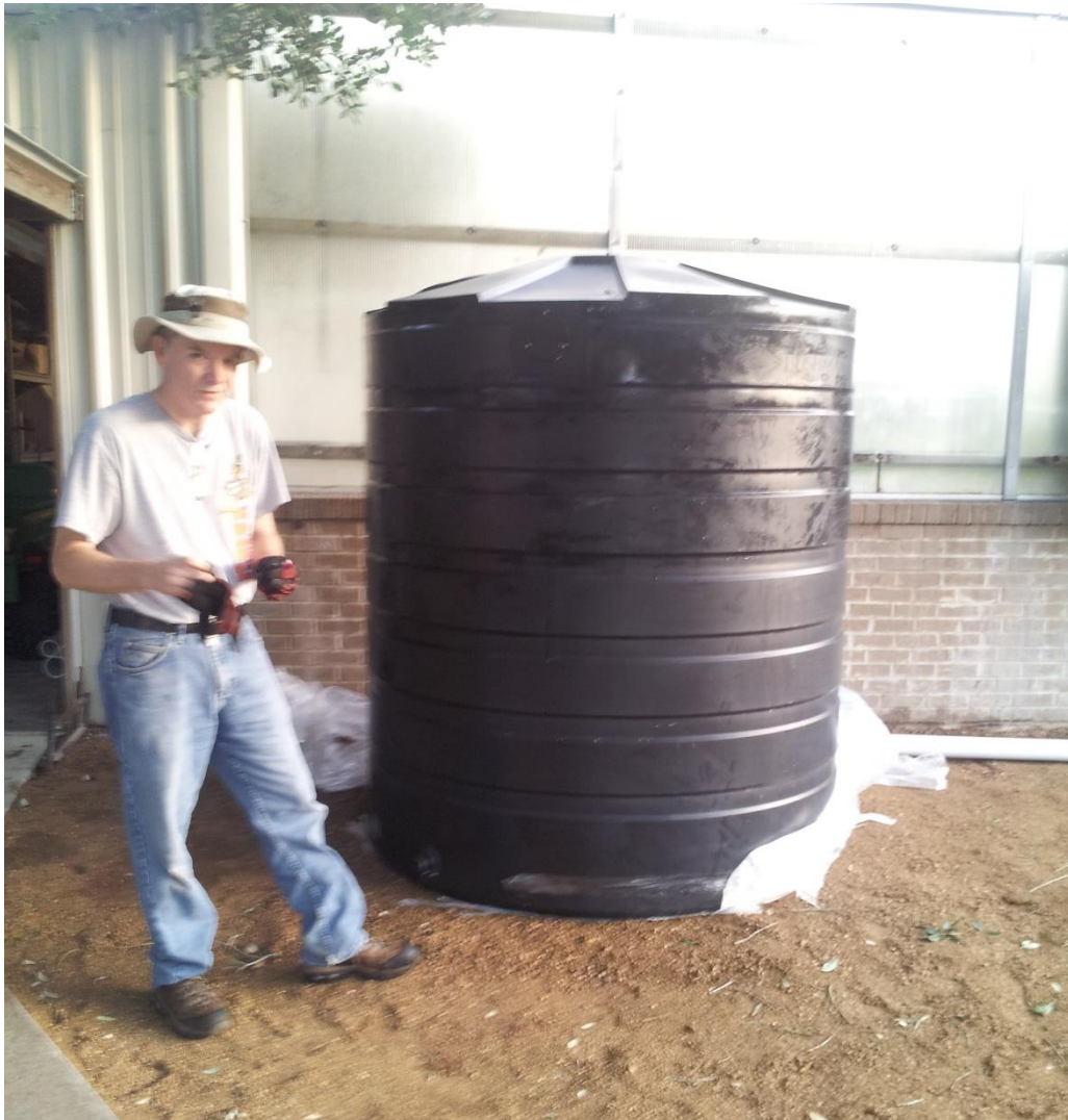
A.2 Example of a 1,000 gallon rainwater harvesting tank (61 inch diameter) at the Harris County Extension Office in Houston (Courtesy: Fouad Jaber)
