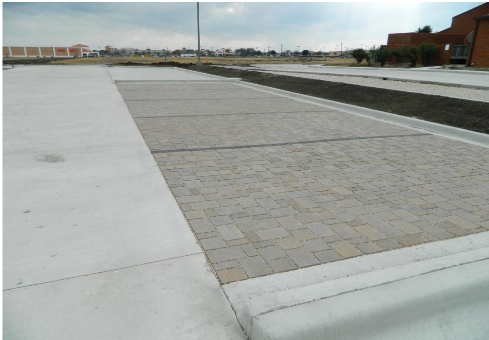
A.3 Example of a permeable pavement (pervious concrete paver (above) and permeable interlocking concrete paver (below) at the Texas A&M AgriLife Research and Extension Center in Dallas) (Courtesy: Fouad Jaber)
