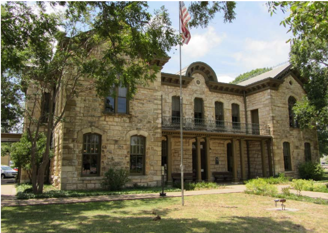
Figure 18. Gillespie County Courthouse, Fredericksburg
