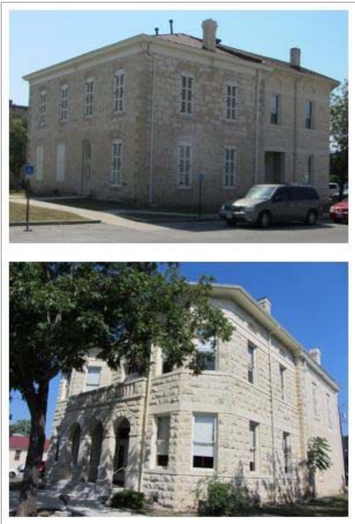
Figure 16. Views of the Kendall County Courthouse, Boerne
