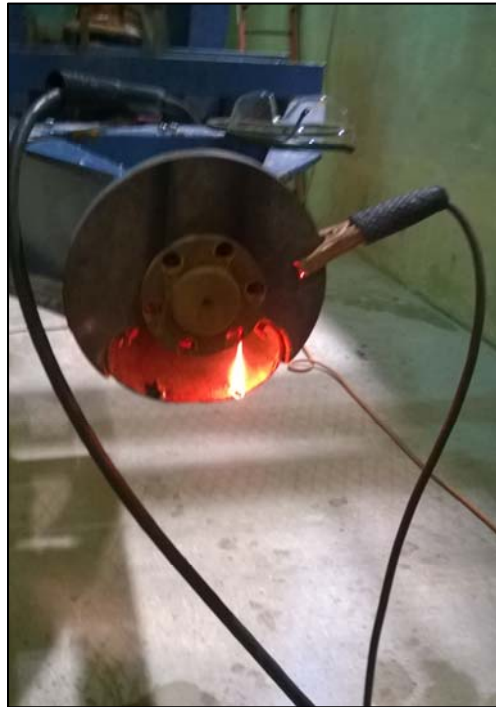
Figure C - 13: Welding bolts to suction mouth.
