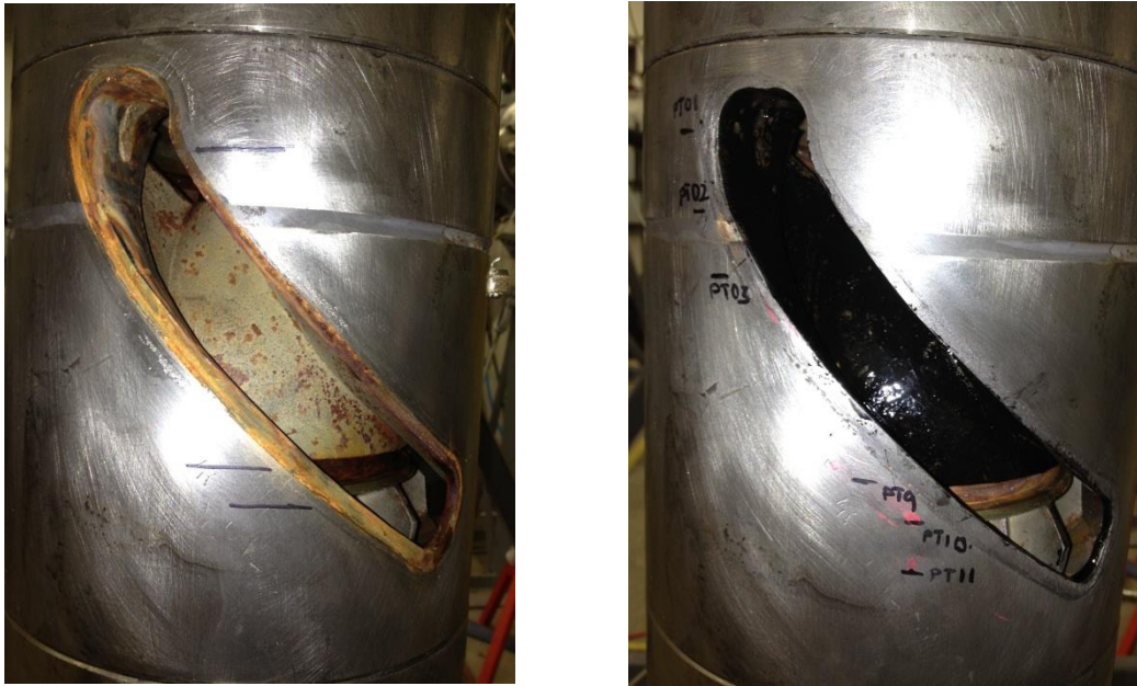
(a) (b) Figure 3-17: Pump's 2 nd stage diffuser (a) before applying insulator paint (b) after applying insulator paint on the non-rotating part of stage. Impellers have been electrically grounded
