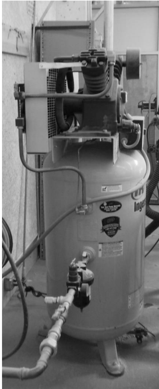
Figure 31. Air Delivery System and Filters
