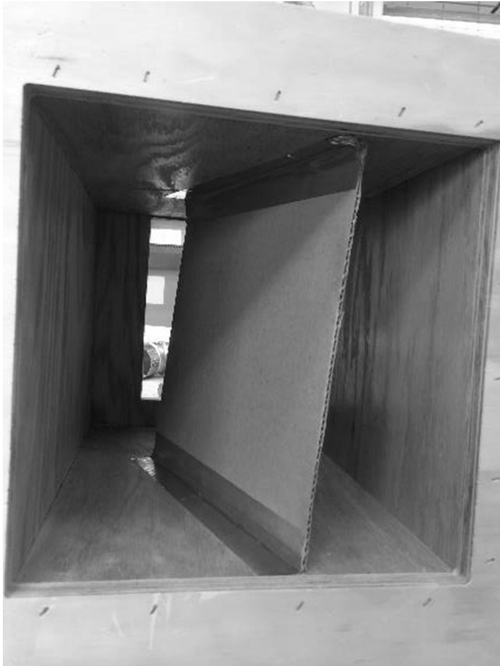
Figure 24. Wall in Containment B Vessel
