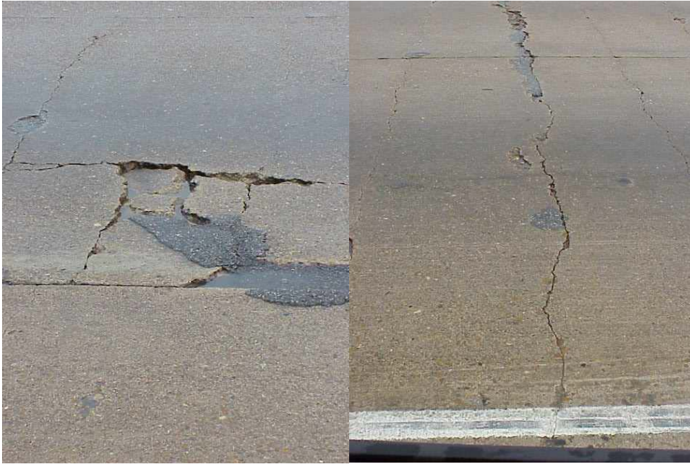
FIGURE 5.4 Distresses in concrete pavements.
