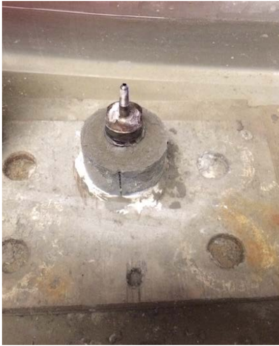
Figure 10: Curing at Surface Conditions
