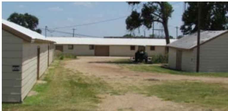
Figure 131 Civil Engineering Maintenance Yard
