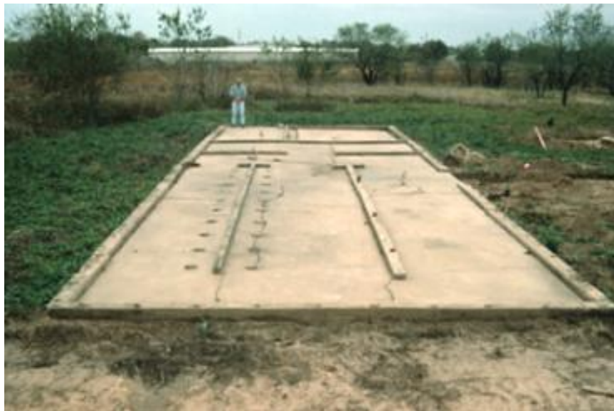
Figure 244 Compound Three Lavatory Foundation (Waters et al. 2006, 236)
