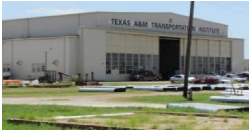
Figure 81 2013 Hanger Two Currently Used by TTI
