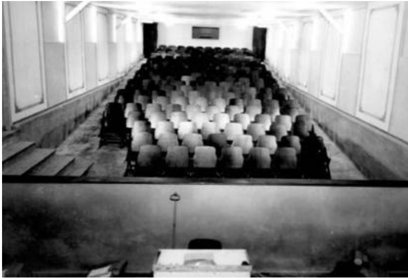
Figure 239 Compound Three Seating Area and Pit in 1944 (Waters et al. 2006, 230)
