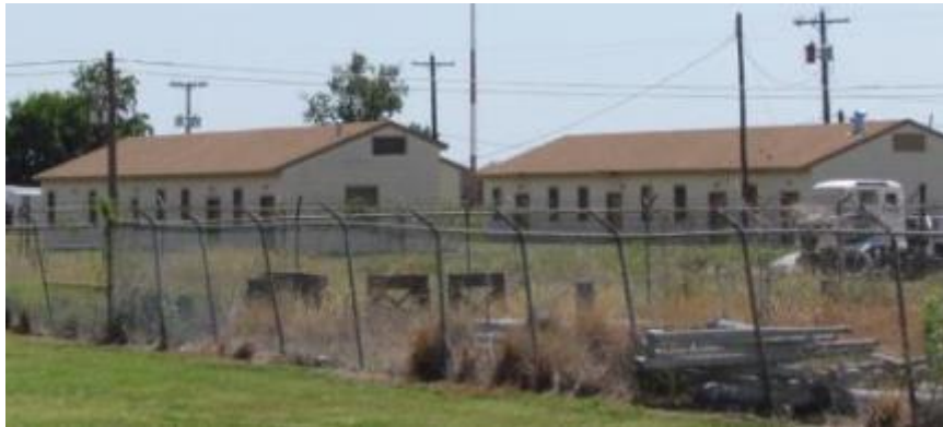
Figure 112 2013 General Purpose Sheds and Shops
