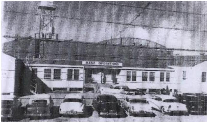
Figure 166 1948 Base Operations Facility (Hankins 2009, 45)
