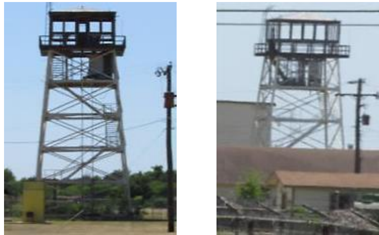
Figure 127 2013 Air Traffic Control Tower
