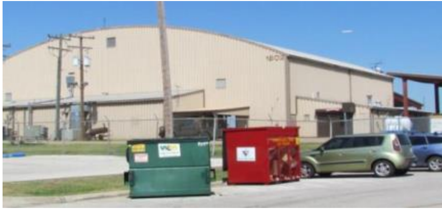
Figure 205 Rear of Building 1602 in 2013
