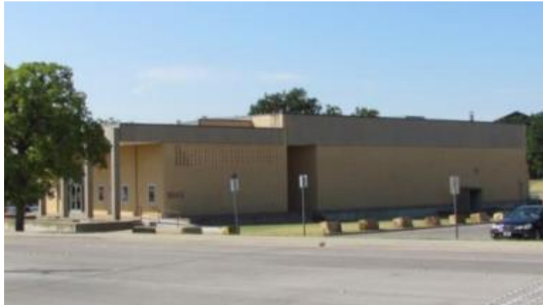
Figure 164 2013 Base Theater Building 1845
