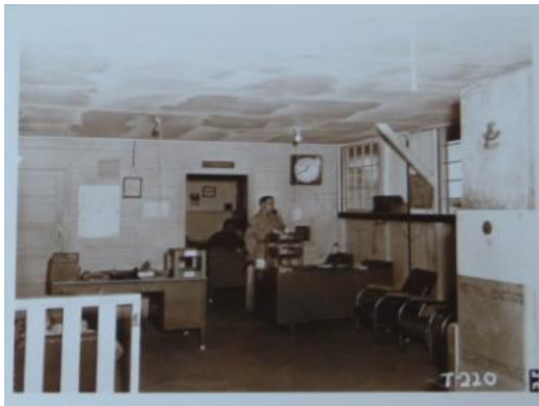
Figure 85 1956 Squadron T-220 HQ Interior
