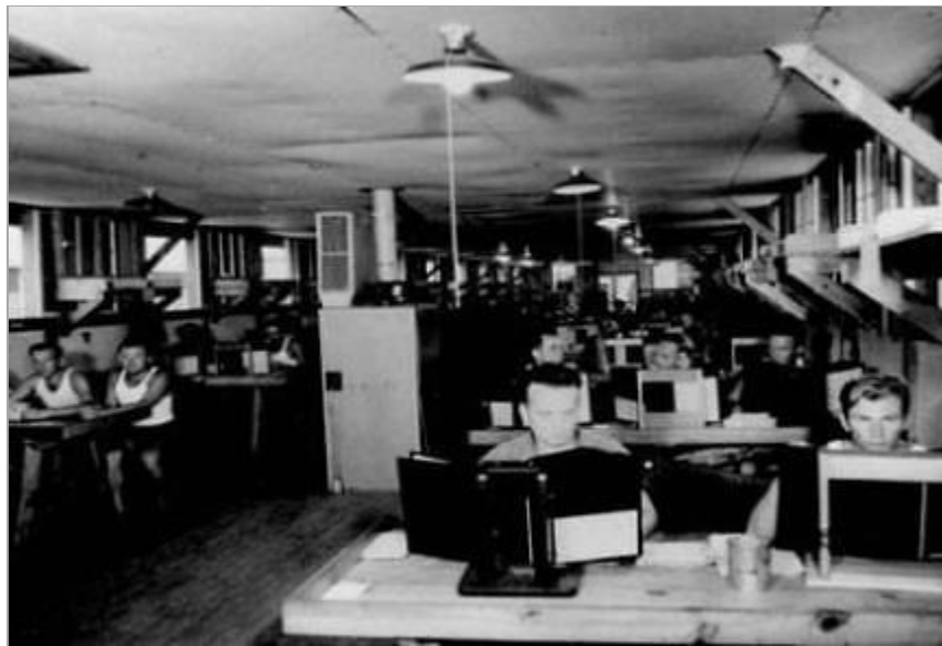
Figure 228 Compound Two POW Post Office (Waters et al. 2006, 98)
