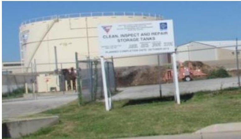
Figure 187 Water Storage Tank near Flight Line
