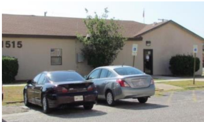
Figure 203 Front Elevation of Building 1515 in 2013
