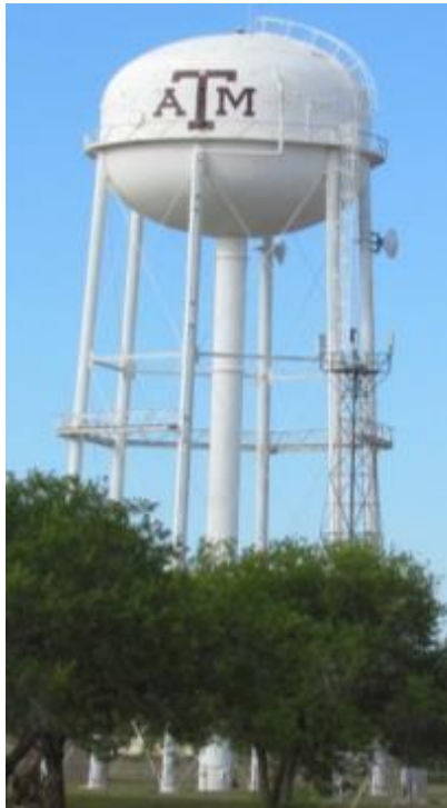
Figure 115 2011 TAMU Water Tower
