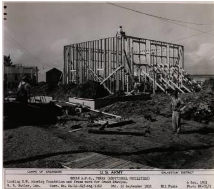
Figure 98 1951 Crash Station Construction
