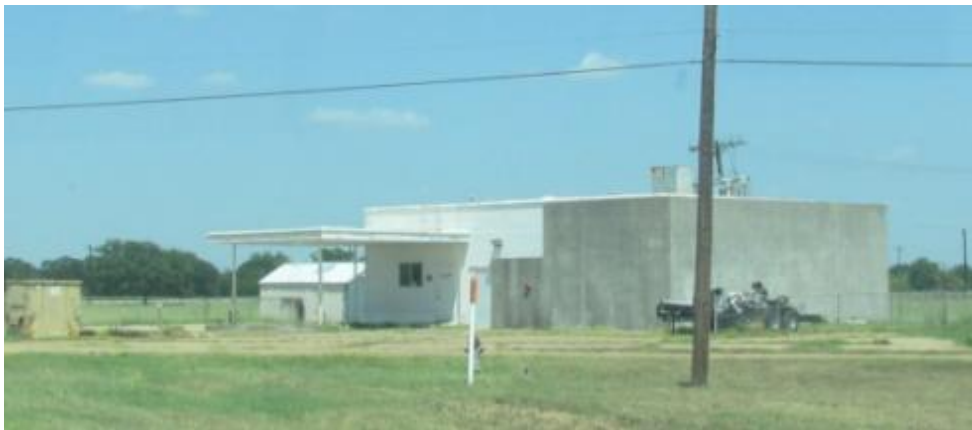
Figure 129 POV Fuel Station in 2013
