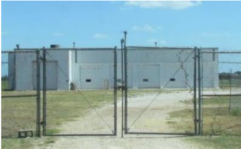
Figure 101 2013 General-Purpose Shop View A
