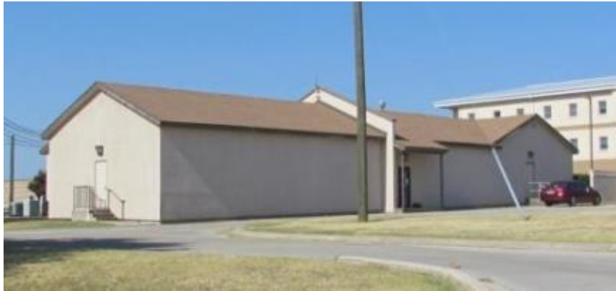
Figure 204 Firewall at Rear of Building 1515
