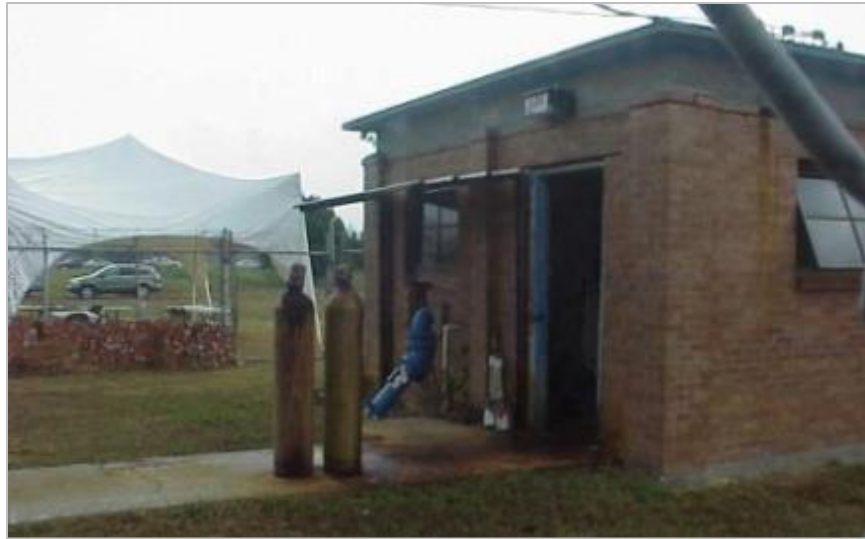
Figure 246 Rear of Original Pump House
