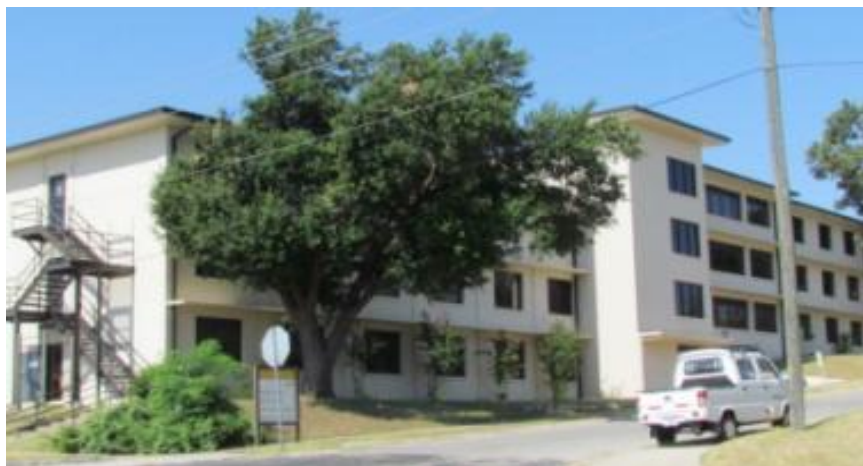
Figure 181 2013 Side Elevation Building 1525
