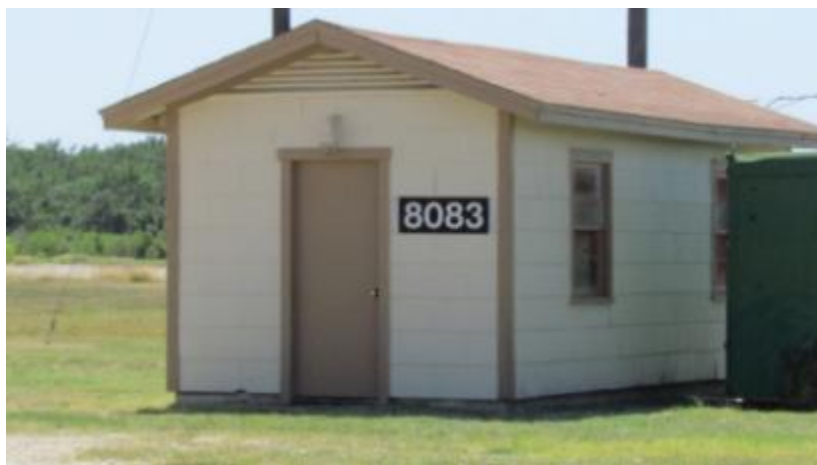
Figure 104 2013 General Storage Building 8083
