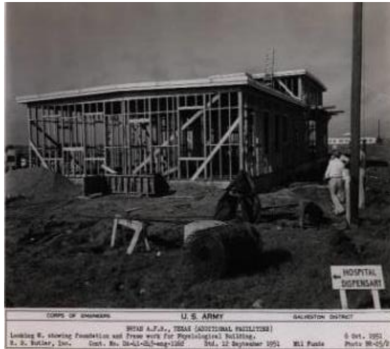
Figure 88 1952 Psychology Building Construction
