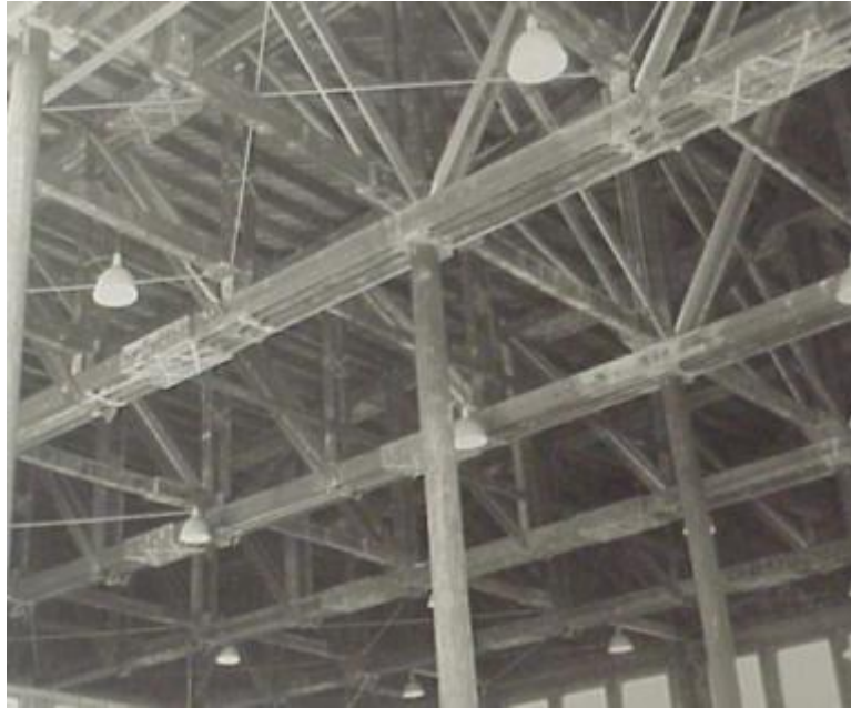
Figure 109 1956 Storage Shed Structure
