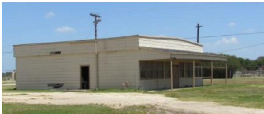
Figure 132 2013 Multipurpose Shop at CE Yard
