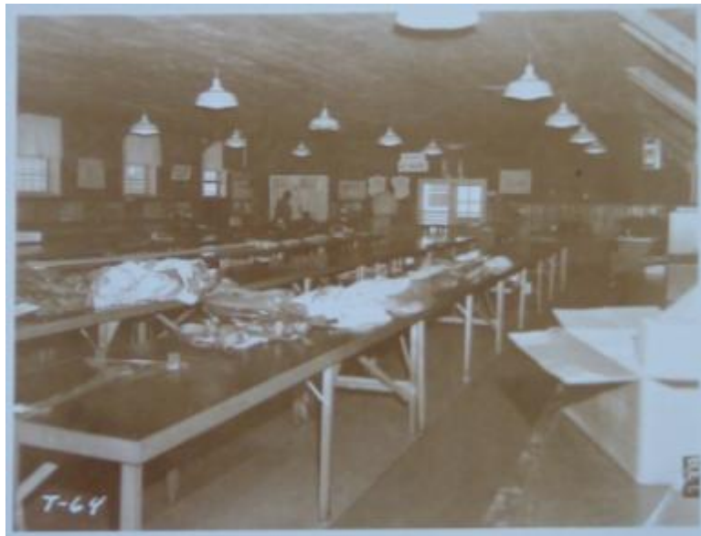
Figure 91 1956 Parachute Shop T-64 Interior
