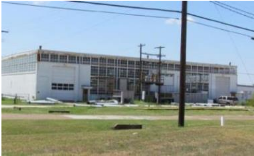
Figure 80 2013 Hanger Currently Used by the TEC
