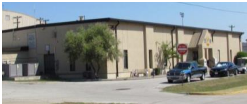
Figure 207 Building 1615 Front Elevation in 2013
