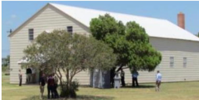
Figure 26 Base Chapel Front View in 2013
