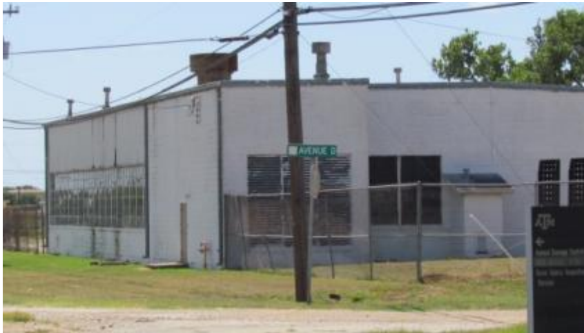
Figure 102 2013 General-Purpose Shop View B
