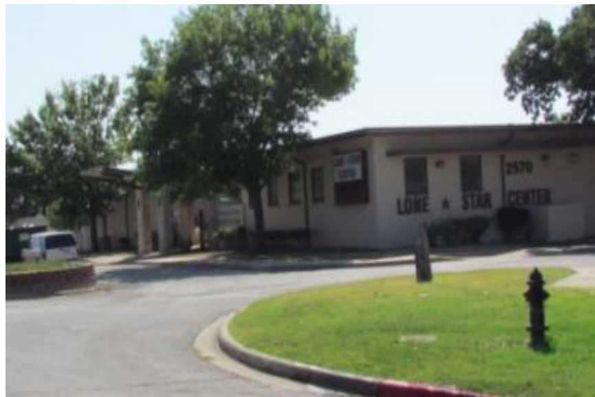
Figure 172 2013 Officers/NCO Joint Club Building 2570
