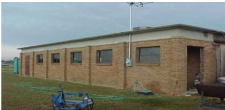
Figure 269 Original Conference Building at Hearne
