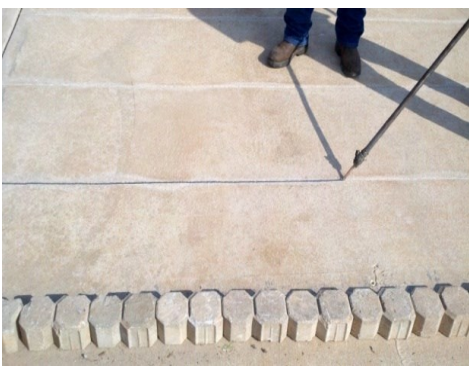
d) Silicon and Hot-pour Placement
