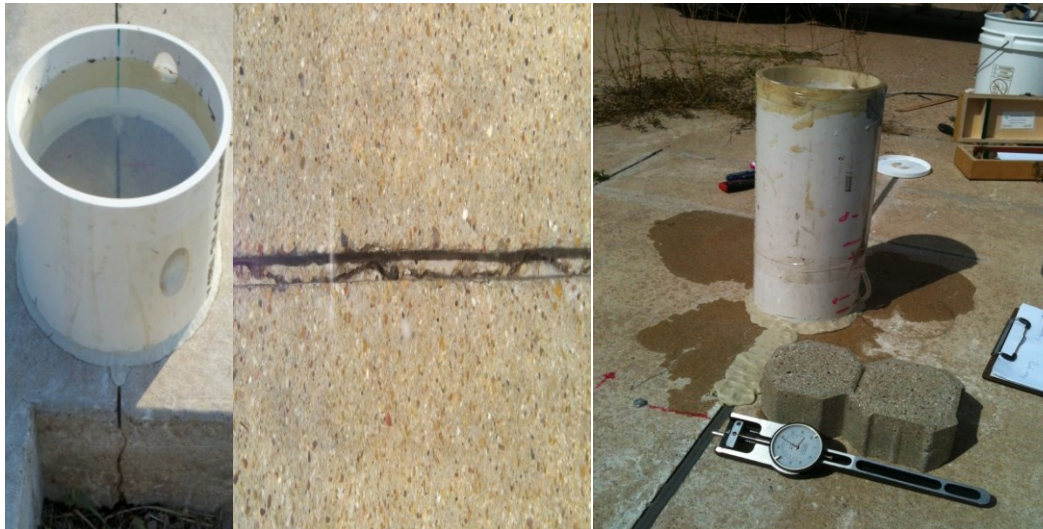
Figure 6 Flow Test on Existing Joint.
