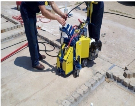
b) Compression Seal Placement
