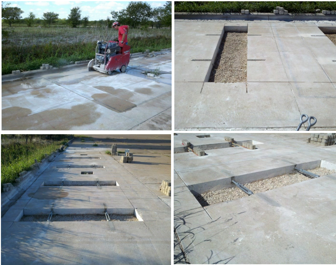
Figure 10 Installation of the Movable Joint System.
