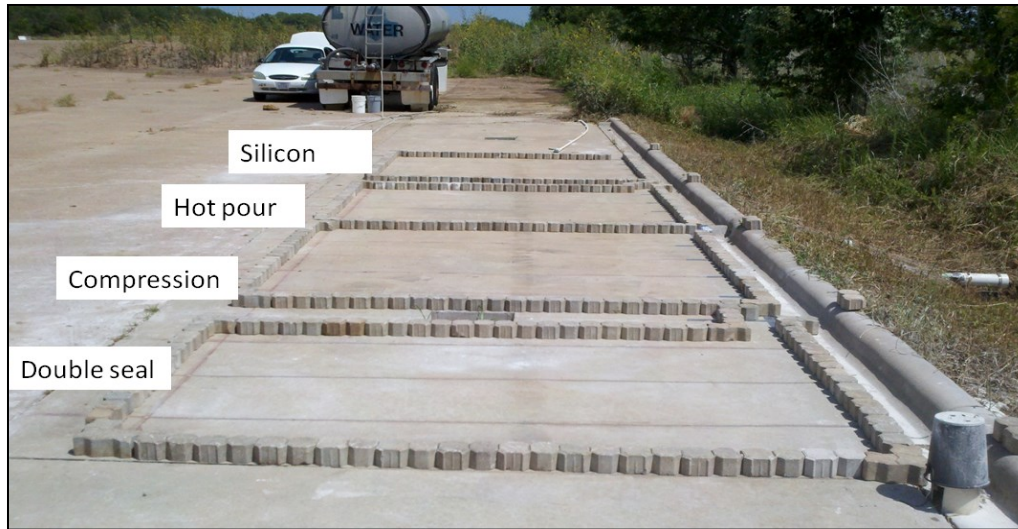
Figure 3 Layout of Joint Sealant Test Area.
