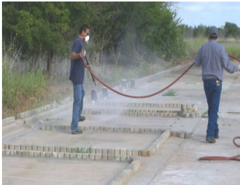
a) Sand and Air Blasting
