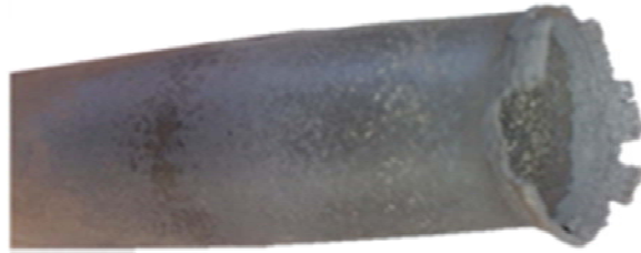
Figure 31 – Melted OFA outlet nozzles
