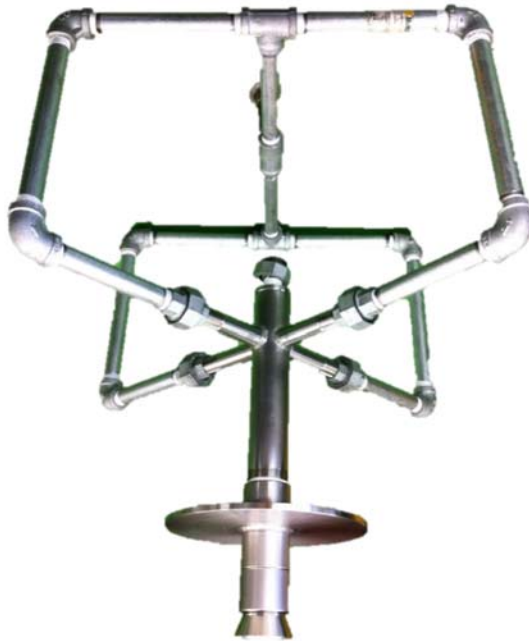
Figure 35 – The modified secondary air piping system attached to the main burner
