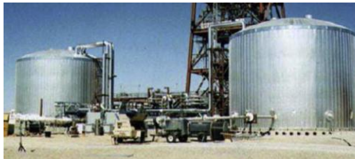
Figure 134: The two-tank storage system of the Solar Two solar plant 16
