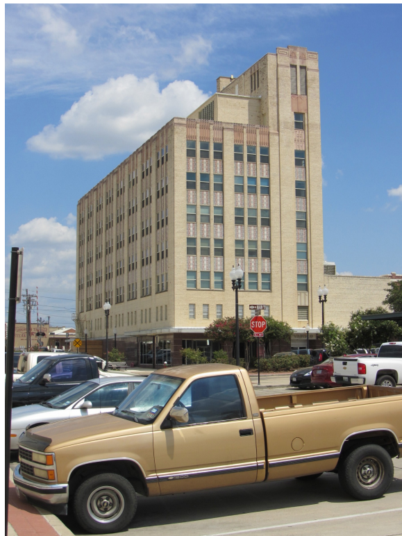
Figure 4. The Varisco Building. Source: Nicholas Samuel
