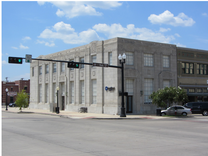
Figure 8. The Former First State Bank and Trust Building. Source: Nicholas Samuel
