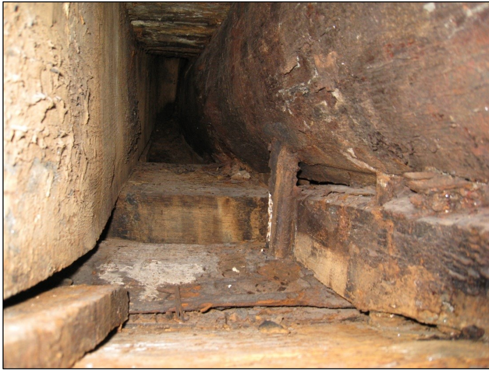
Figure 3.7. Photograph taken in between two of Vasa 's floor timbers. The tingel (a wedge-shaped timber filling in the space between the garboard and the keel) and chocks can clearly be seen – filling in space left by roughhewn floor timbers. Also visible is the unfinished surface of the floor timber on the right and a carelessly placed treenail. Photograph by Kelby Rose.
