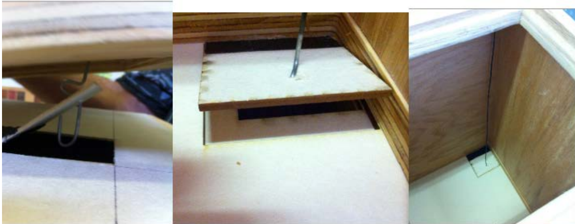
Figure 15. Complete work of door on the barrier
