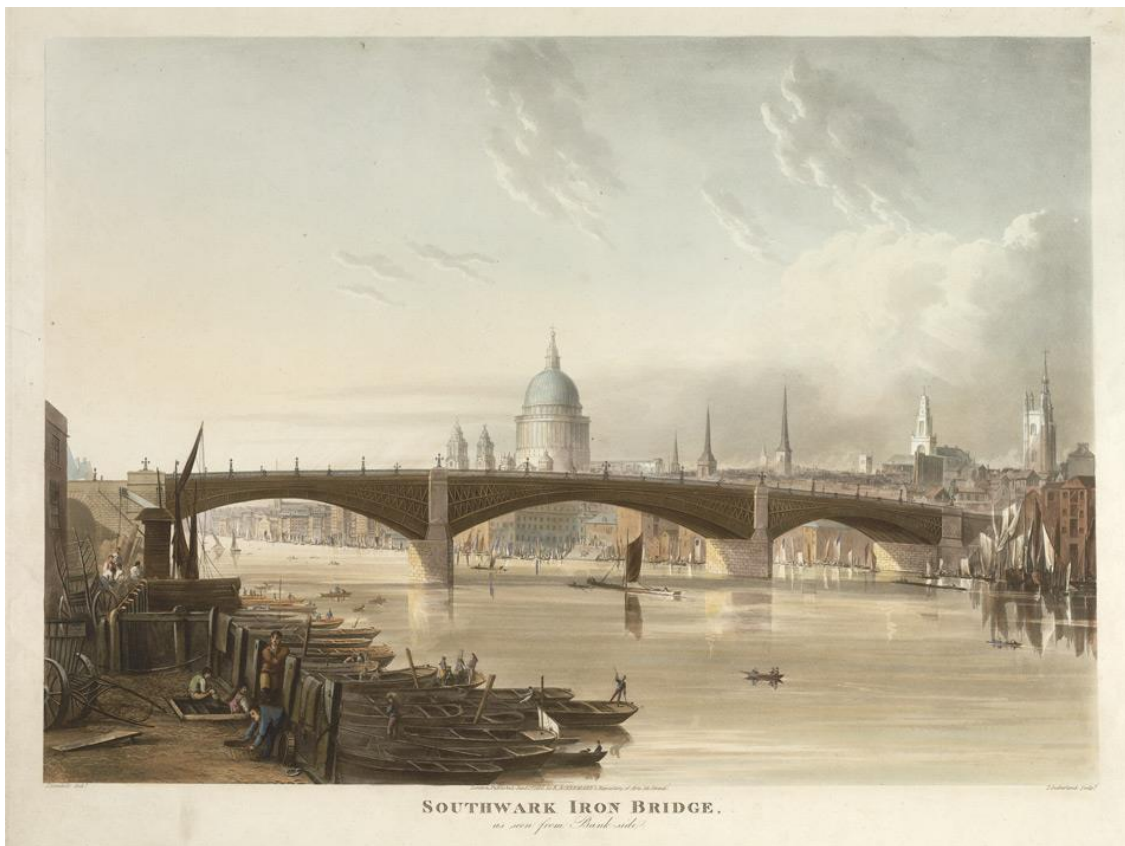
Figure 50. Southwark Iron Bridge, as seen from Bank-side, by Sutherland, T., 1818
