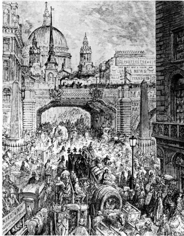
Figure 58. London, Ludgate Hill viaduct, engraving by G. Doré 1870 (Benevolo, 1971, p. 143)
