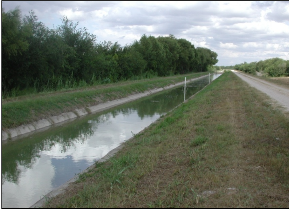
Figure 3. Raised concrete lined canal with supporting levees.
