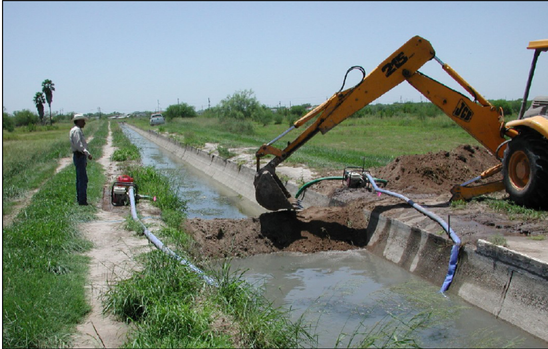
Figure 5. Earthen dam being built by backhoe (Leigh and Fipps 2008c)
