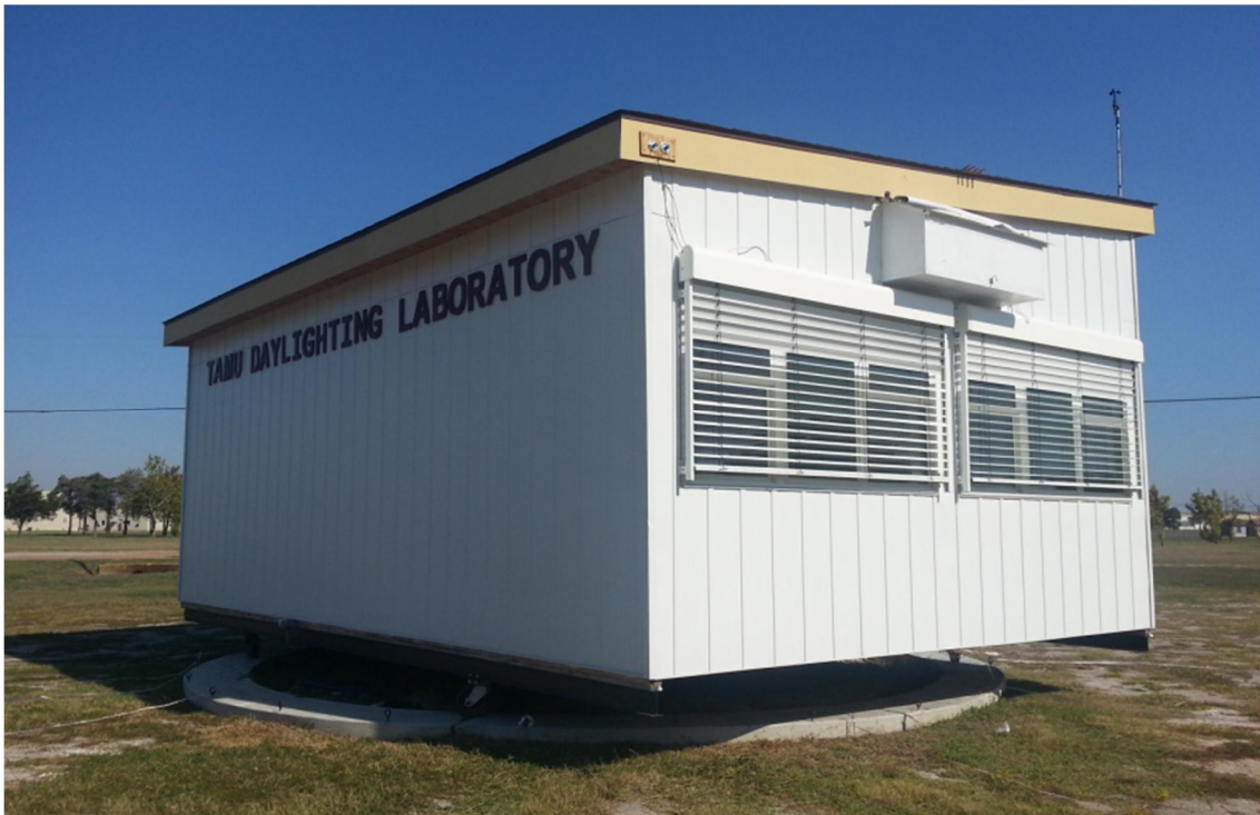
Figure 4.1. Exterior view of the mockup test structure
