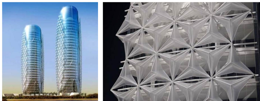
Figure 2.8. Al Bahar Towers and the kinetic sunscreen (Cilento, 2013)
