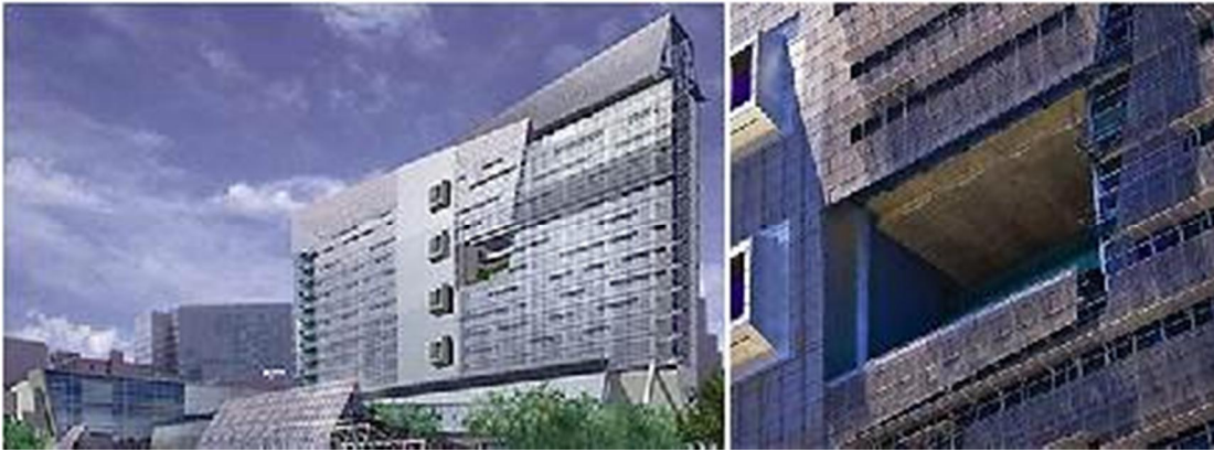
Figure 2.15. The double skins of the San Francisco Federal Building (Morphosis, 2011)
