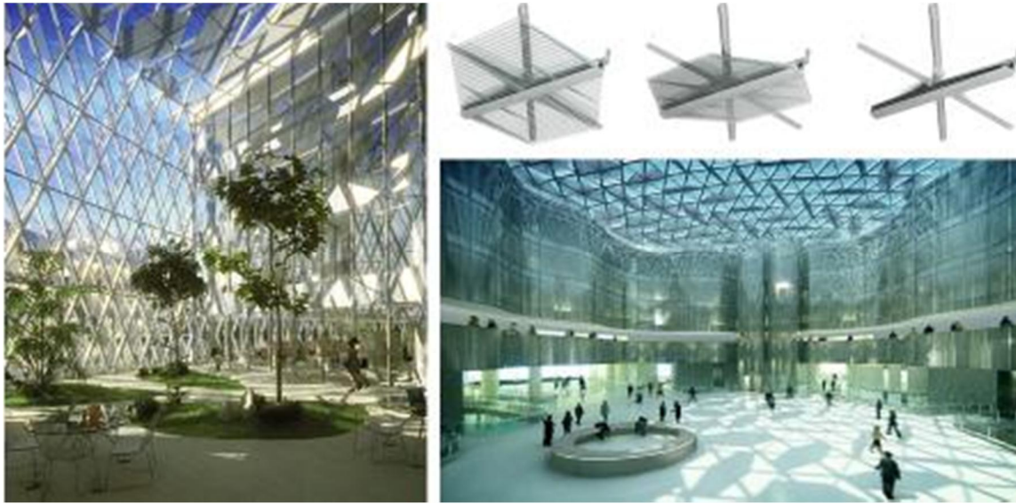
Figure 2.11. Retractable roof of the High Court of Justice and Supreme Court (Foster+Partners, 2012)
