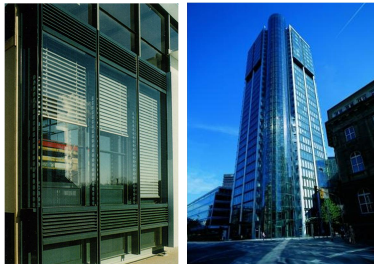
Figure 2.7. Eurotheum and the motorized blinds between the double skins (Hertzsch, 1998)
