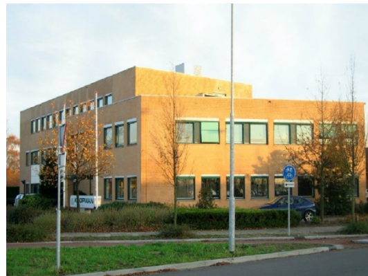
Figure 2: Test case office building Kropman Breda.
